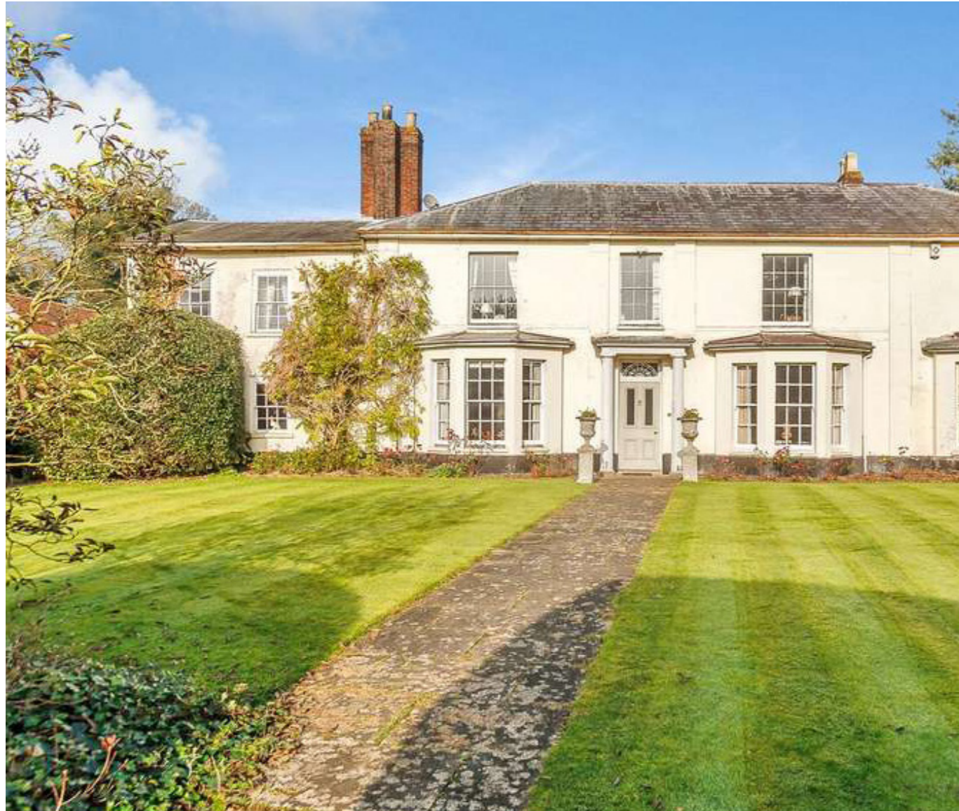
Above: Photograph of existing front facade and front garden of Turville Heath House
