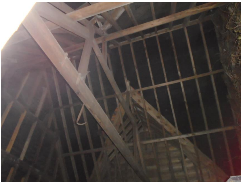
West end interior / roof
