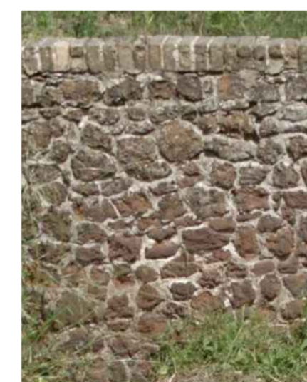
EXISTING CARRSTONE WALL
