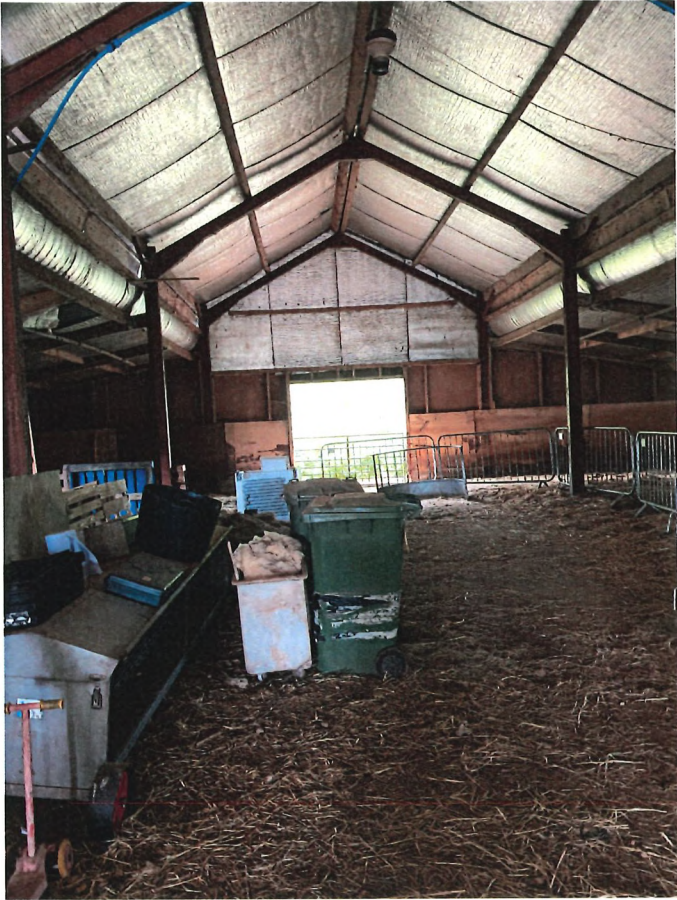
Barn at Green Hill Farm, Dymock, GL18 2AD
