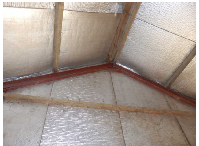
Photo 7. Under side of roof and inner side of western elevation.
