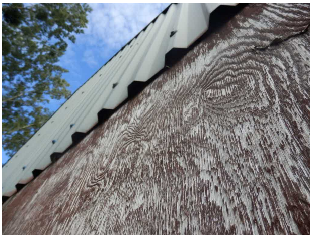
Photo 4. Gap between metal and plyboard
