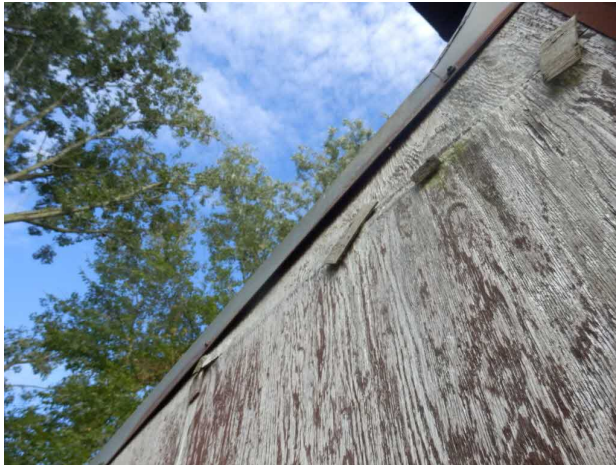
Photo 6. Weather boarding on north gable
