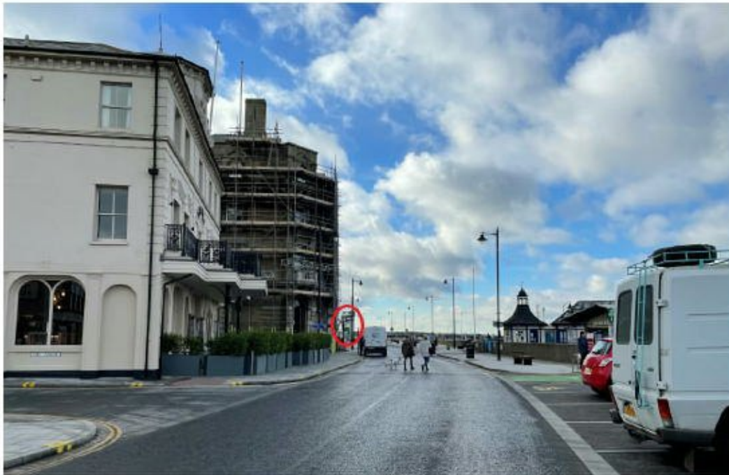
Figure 16 View from the northern-eastern end of the Quay towards the Train Ferry Gantry
