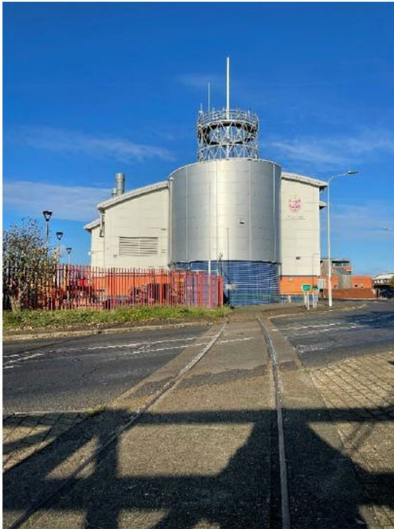
Figure 14 Railway approach and Trinity Buoy shed
