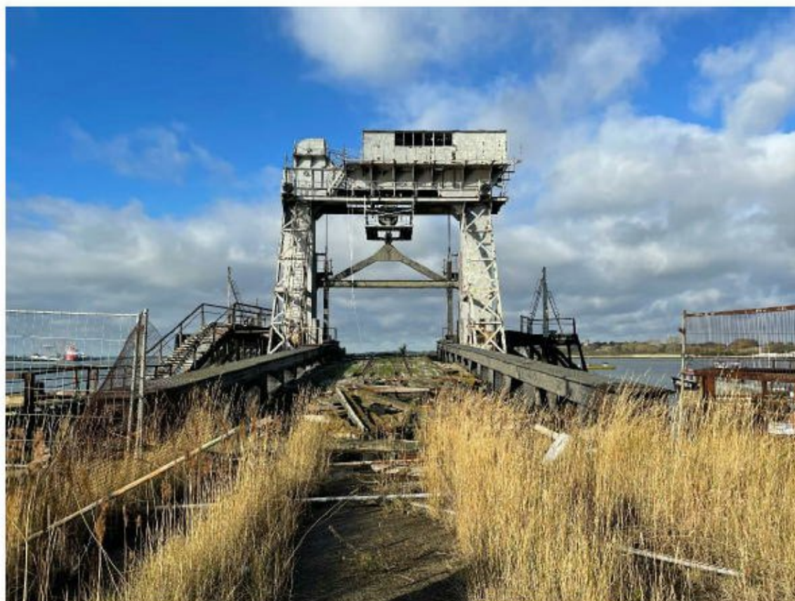
Figure9 The Train Ferry Gantry from the concrete approach
