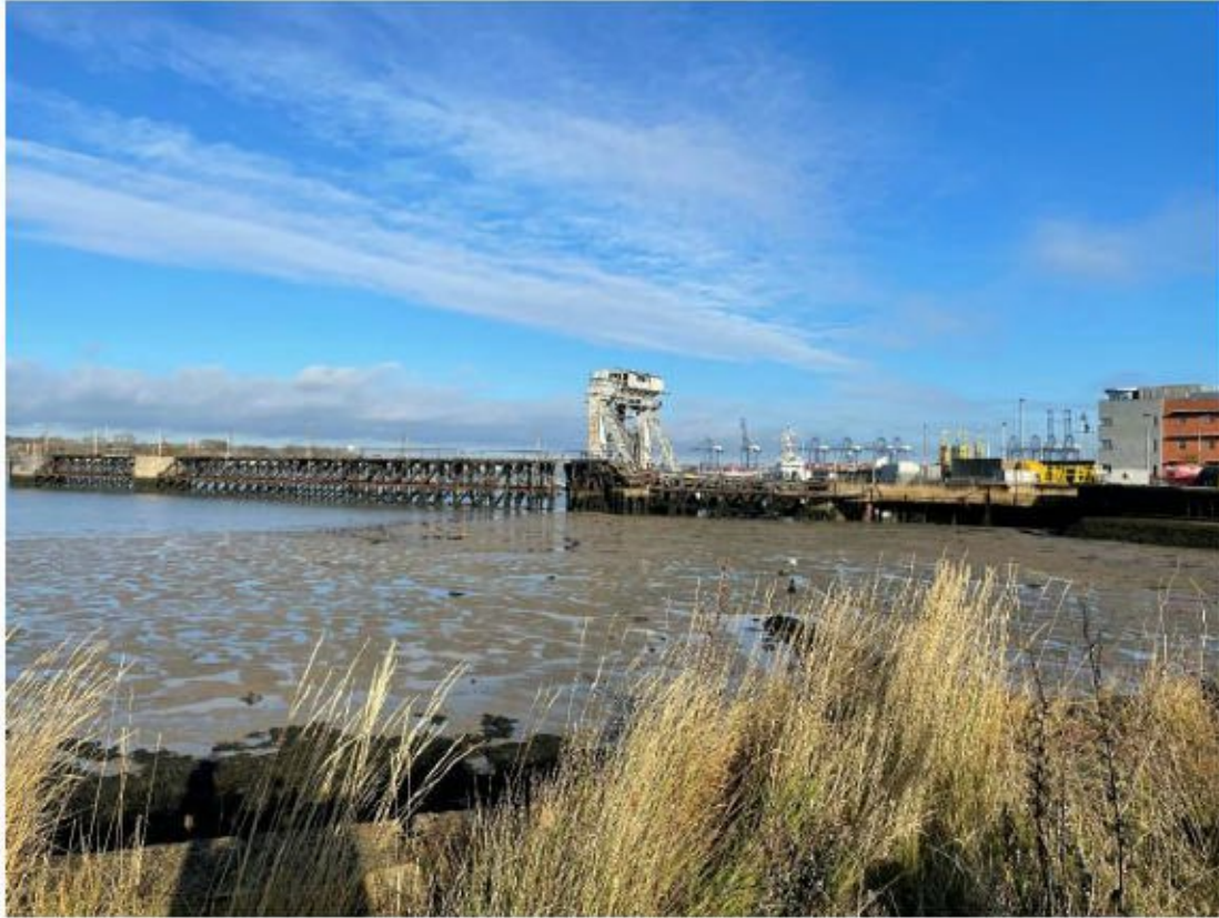
Figure 10 The Train Ferry Gantry including the long berthing arm from the approach to Harwich
