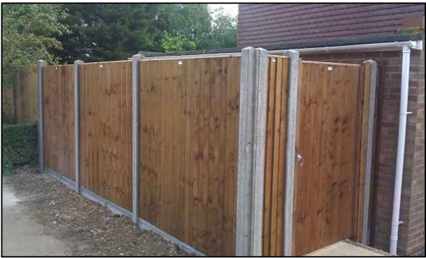
Example of 1.8 Metre high closeboard fence with concrete posts and concrete gravel boards.
