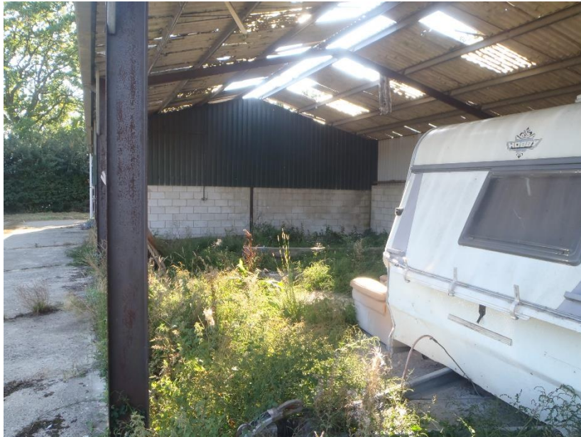
7. Barn Bays 1 to 3
