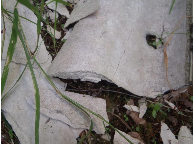
11. Roof Sheet Cement in Bay 1
