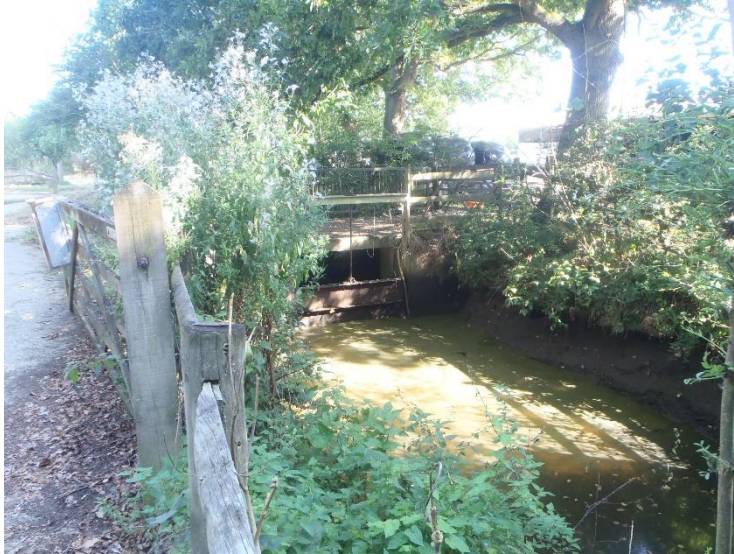
1. Sluice Gate on Southern Boundary
