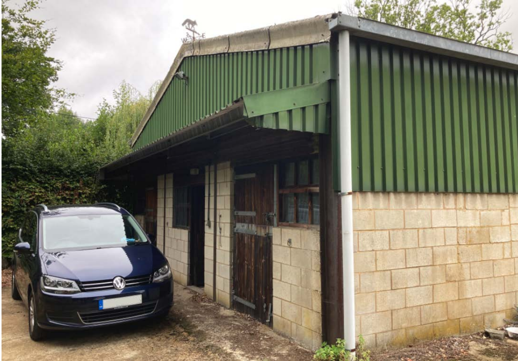
Fig 5 View of the existing building
