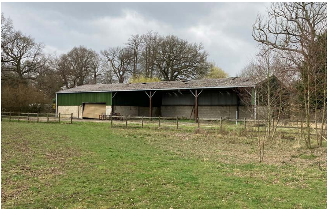
Fig 4 View of the existing building from within the site
