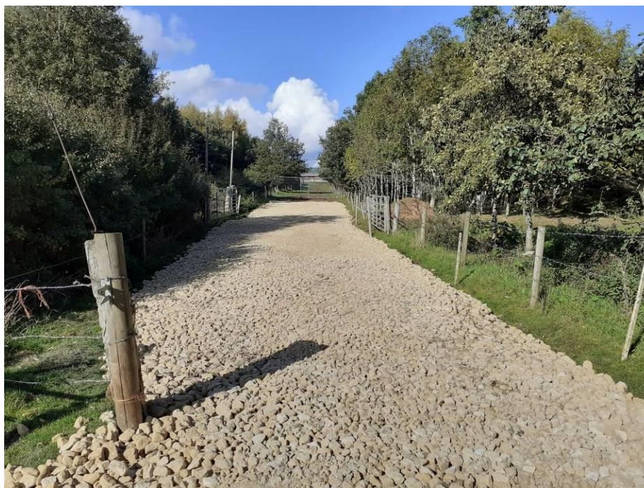
Figure 2. Example of recently resurfaced track using same hardcore resurfacing methods
