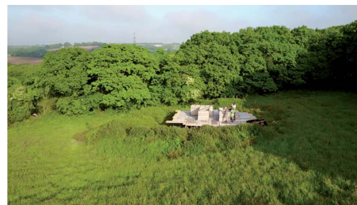
management of waterways and removal of redundant structures
