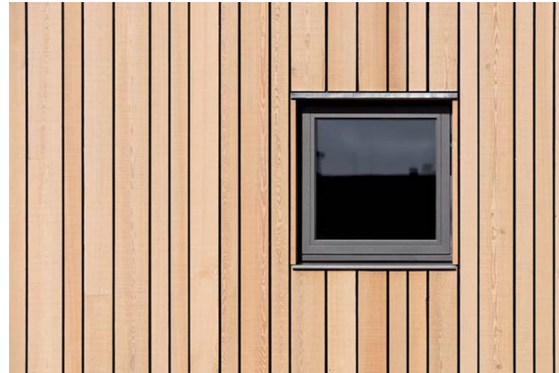
Timber Cladding - random width vertical pattern
