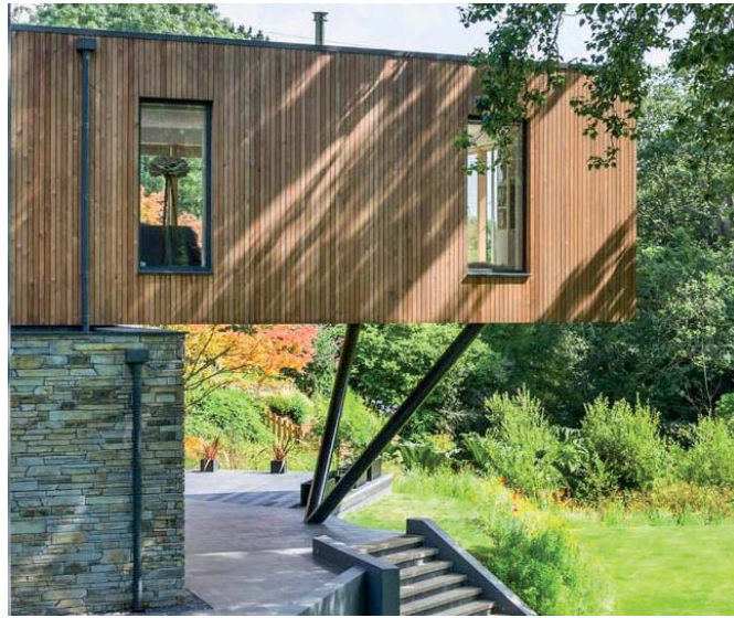
Examples of natural stone, aluminium windows and timber cladding combination
