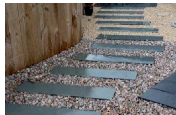
natural permeable paving
