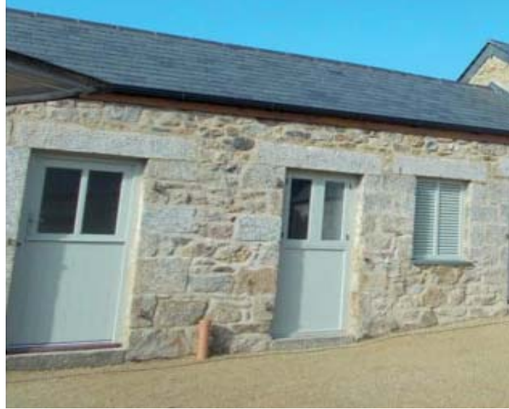
Natural stonework with painted timber doors, slate roofs and slate verges for the historic mill and cottage
