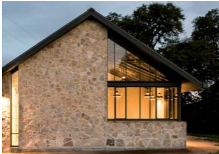
Natural stonework with painted timber doors, slate roofs and slate verges for the historic mill and cottage
