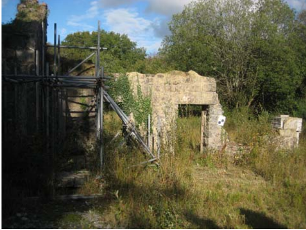
Brynn Mill and Cottage Existing Stone wall made safe and stabilised
