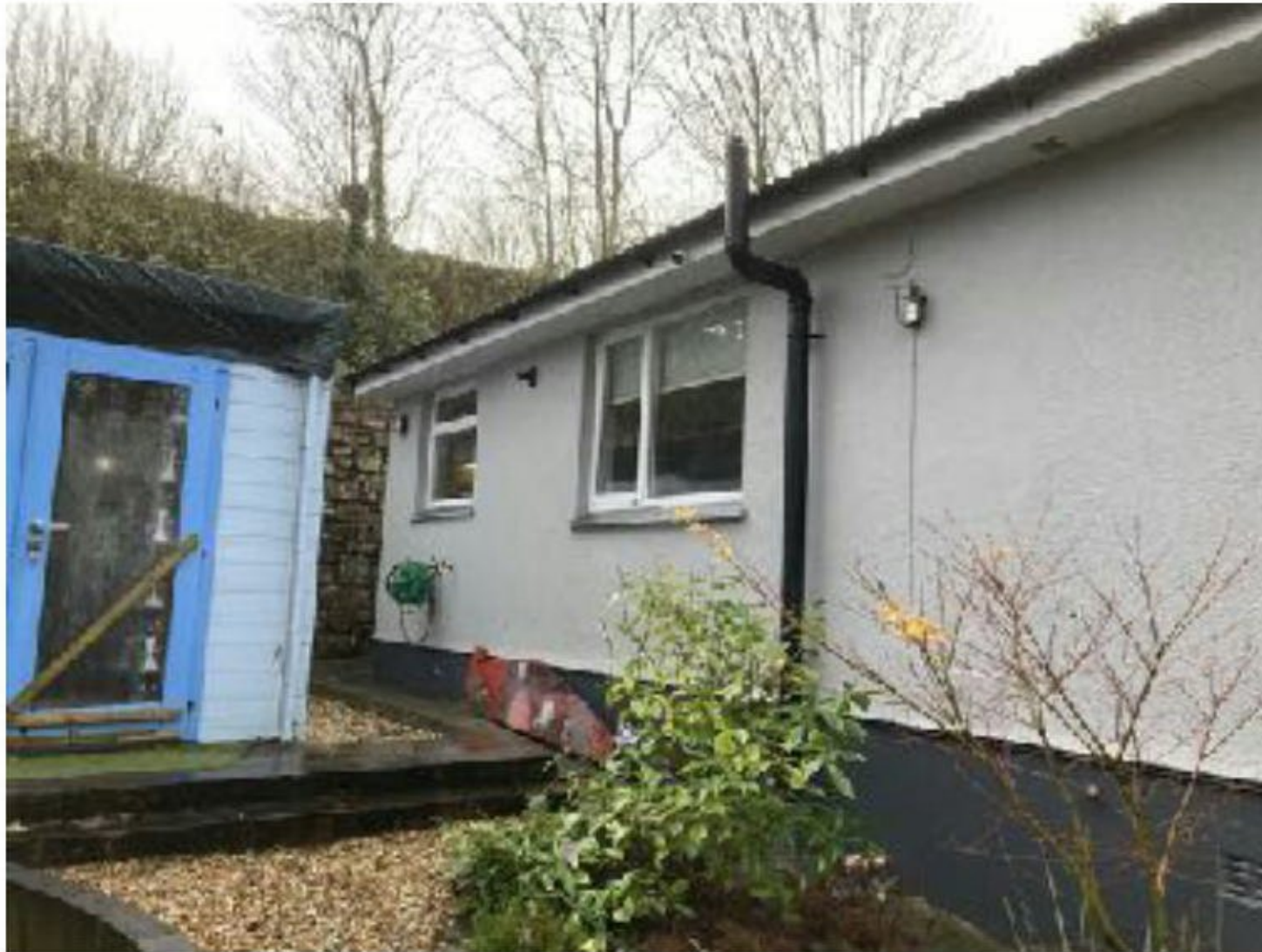
The site of the proposed extension which will replace the existing garden room.
