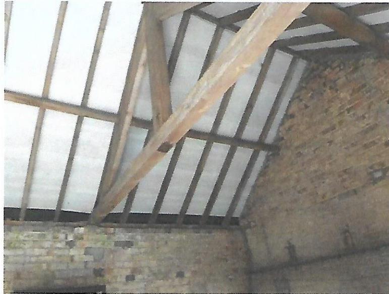
Photograph 11: Interior of main barn with lined, intact membrane
