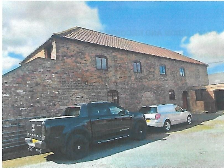
Photograph 1: Exterior view of the barn roof, showing intact pantiles
