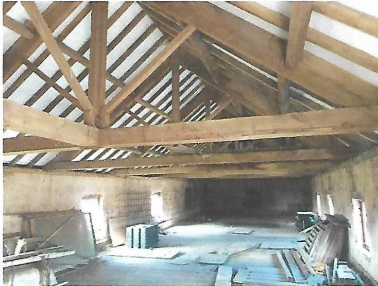
Photograph 3: General view of barn roof internally, showing intact membrane
