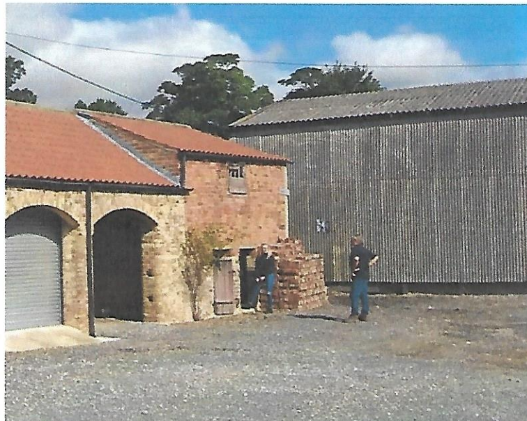
Photograph 12: Exterior view of the dovecote which shows intact pantiles
