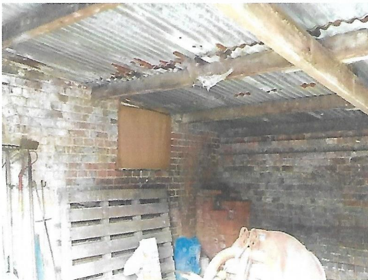
Photograph 10: Ancillary building with corrugated roof
