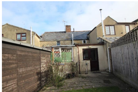
2. 3 Bell Lane from the rear (right-hand property)
