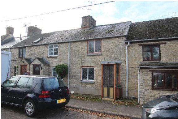
1. 3 Bell lane (left with stone porch) from NW
