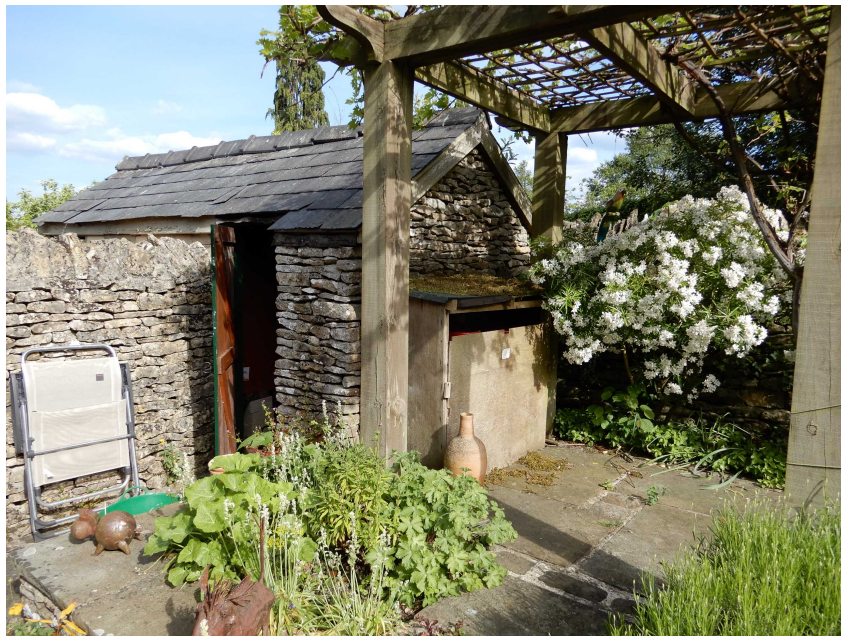
REAR VIEW OF FLORA COTTAGE STONE SHED
