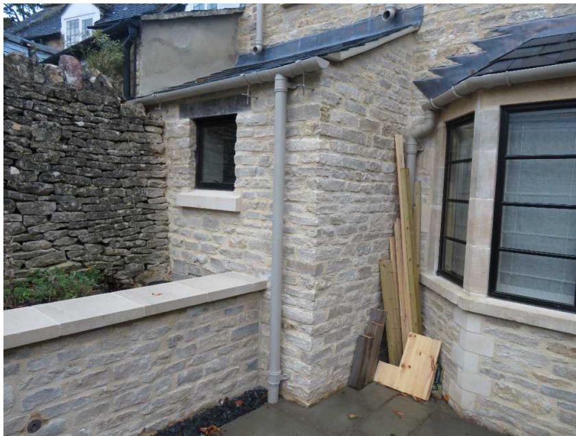
BOUNDARY WALL BETWEEN JASMINE COTTAGE AND FLORA COTTAGE
