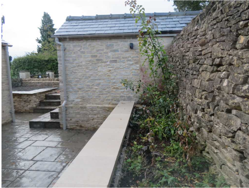
REAR VIEW OF JASMINE COTTAGE OUTBUILDING AND BOUNDARY WALL
