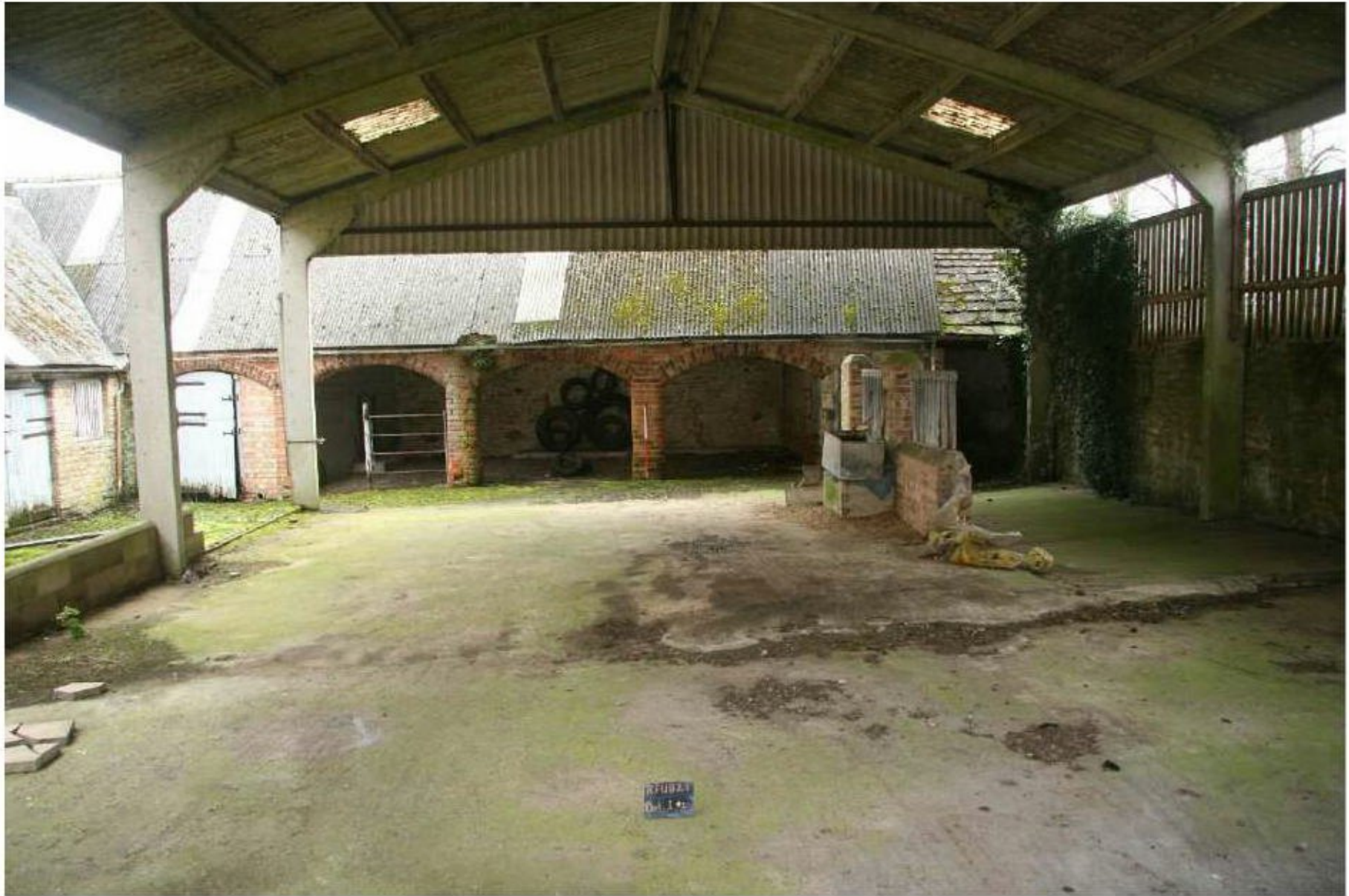
Plate 1: Building A elevation 1.
