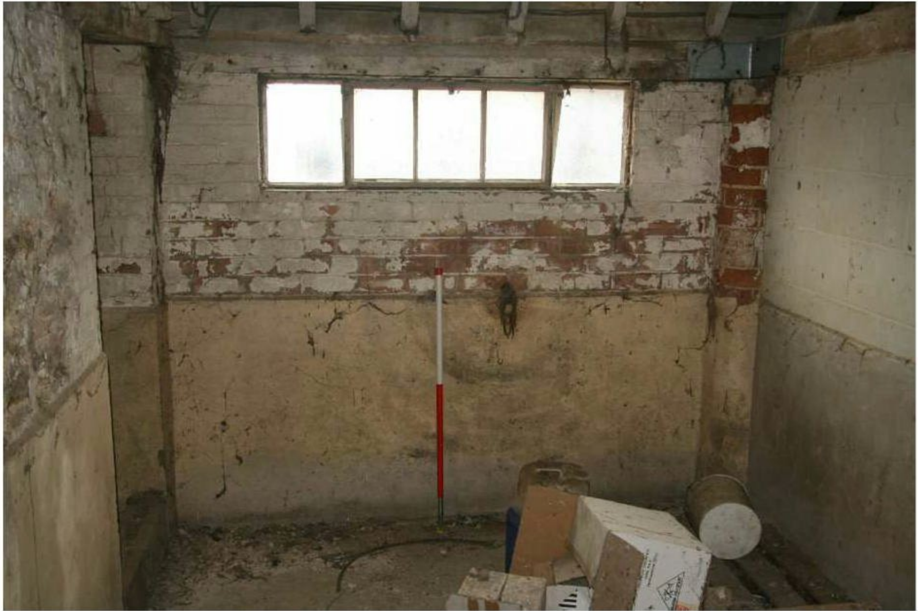
Plate 31: Building F, western room, looking northwest
