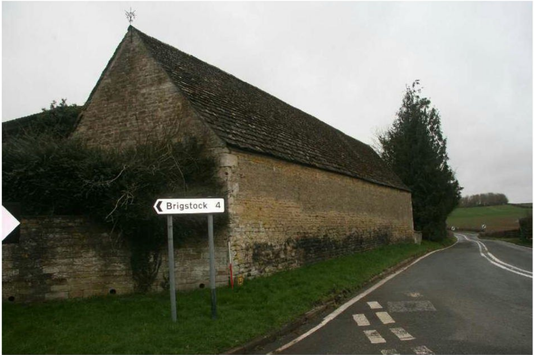
Plate 7: Building A and B elevation 2, looking southwest
