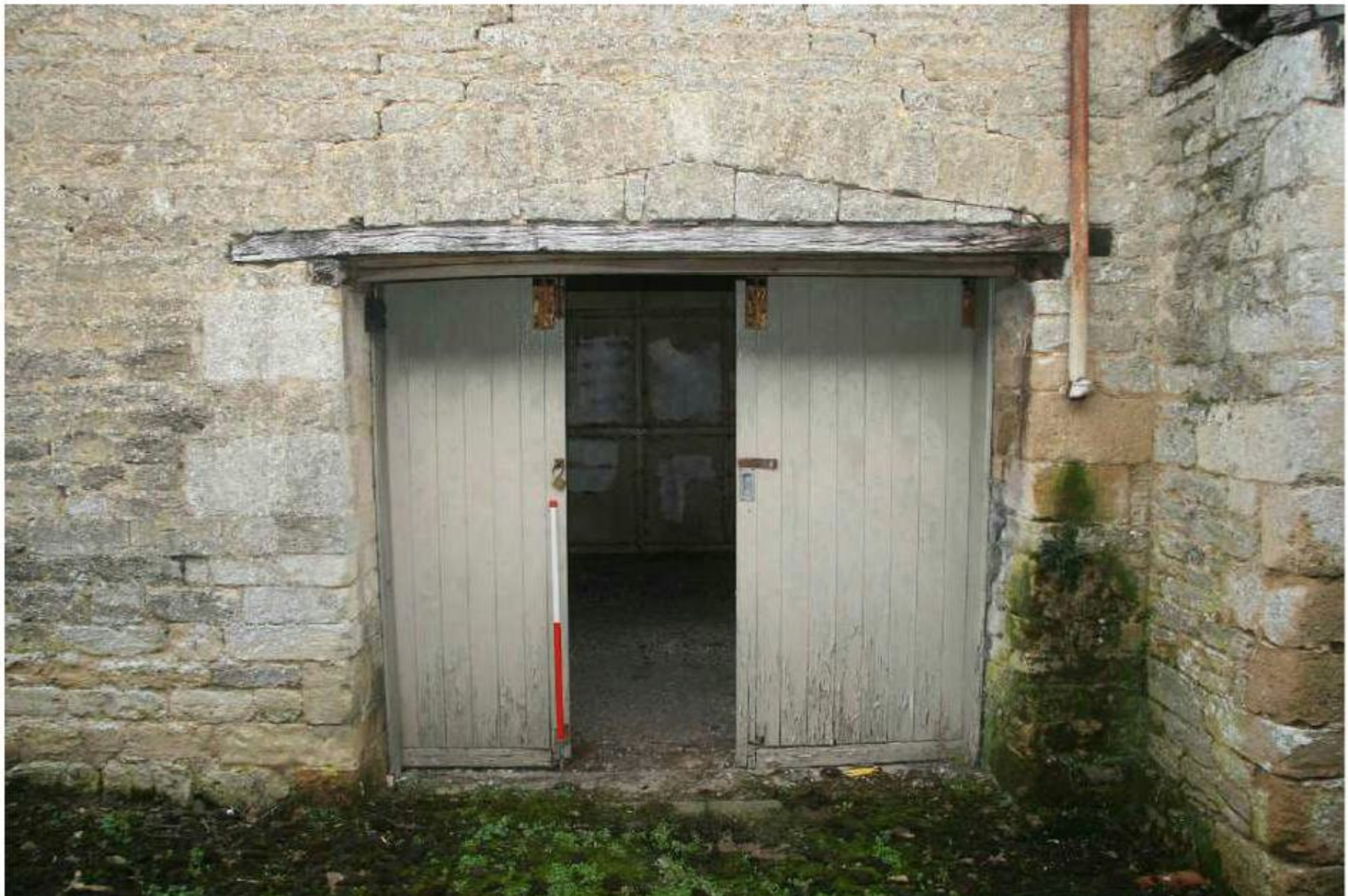
Plate 20: Building D, elevation 3, looking northwest.
