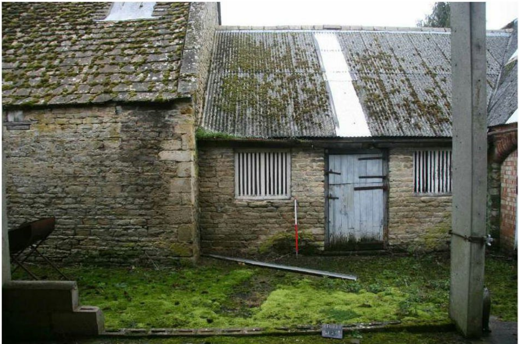
Plate 12: Building C and D elevation 2, looking north.
