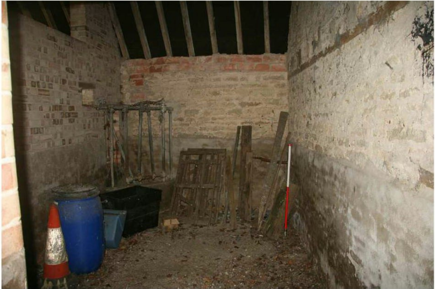
Plate 3: Building A, southern room, looking east
