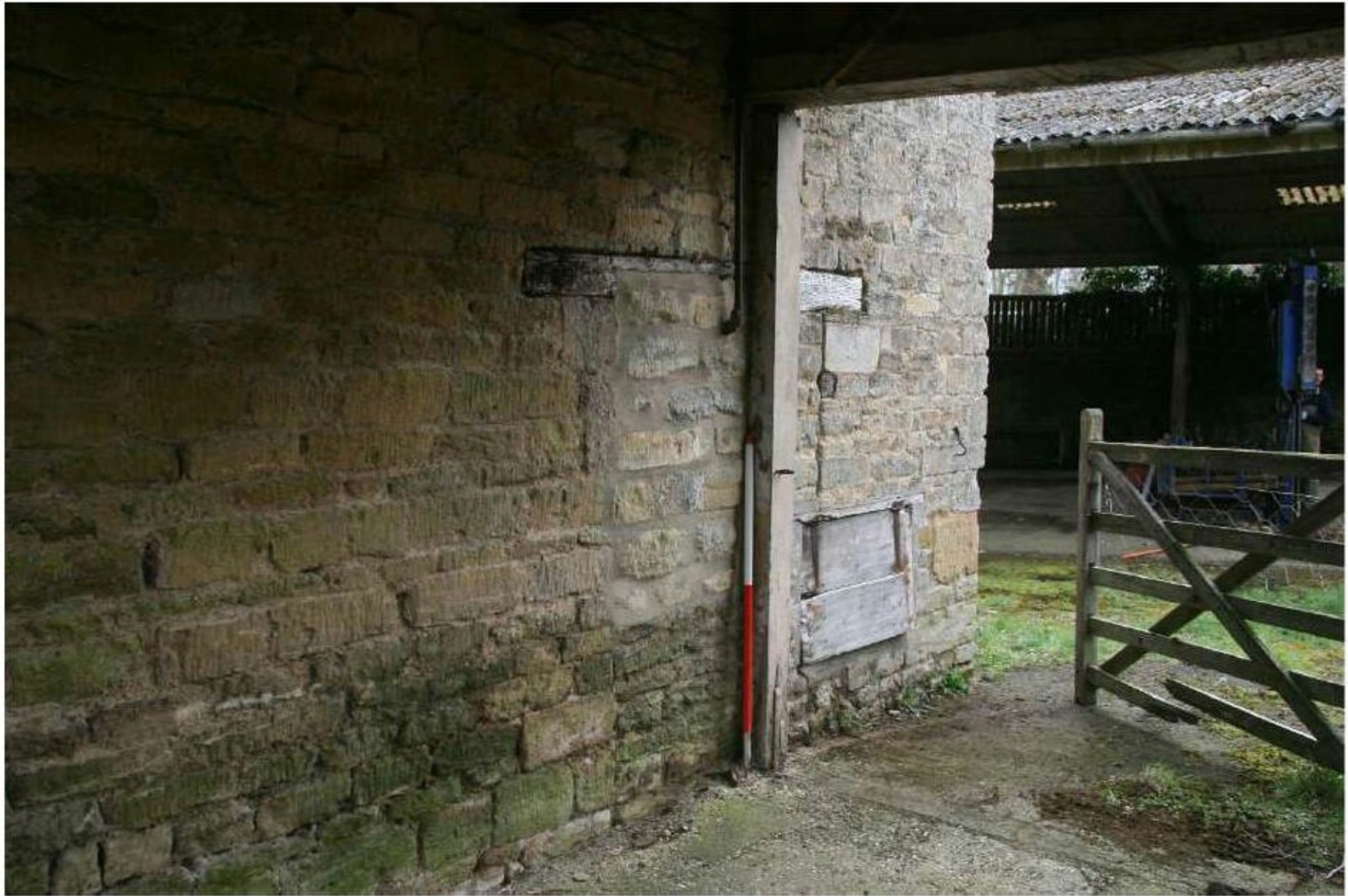
Plate 21: Building D, looking northeast
