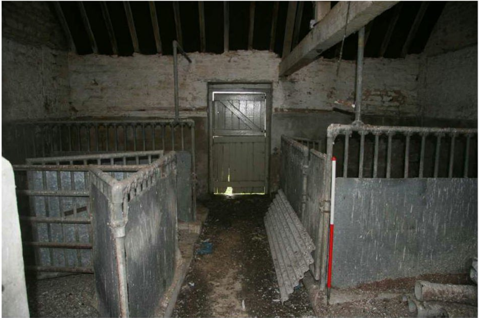
Plate 11: Building C, looking north.
