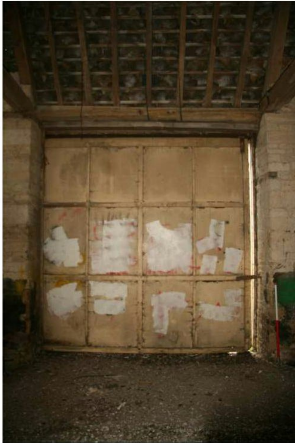
Plate 19: Building D, looking northwest.
