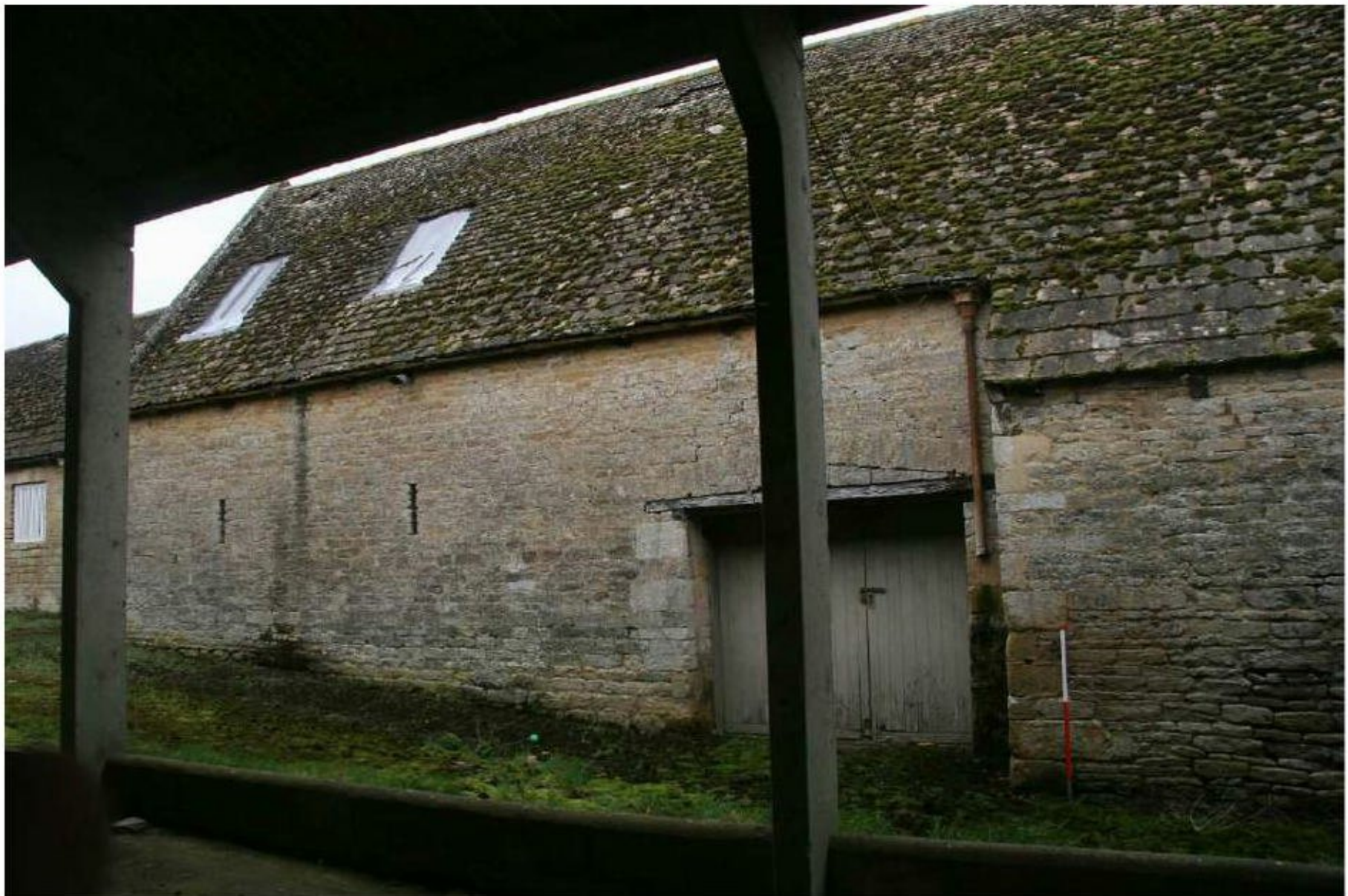
Plate 14: Building D, elevation 3, looking northwest.
