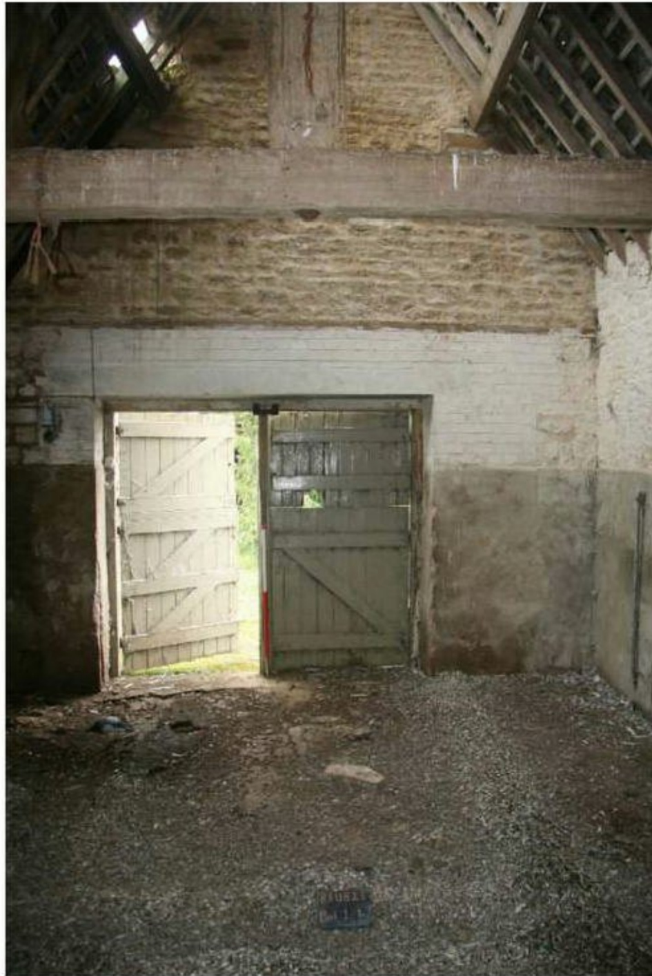
Plate 9: Building B, looking north.
