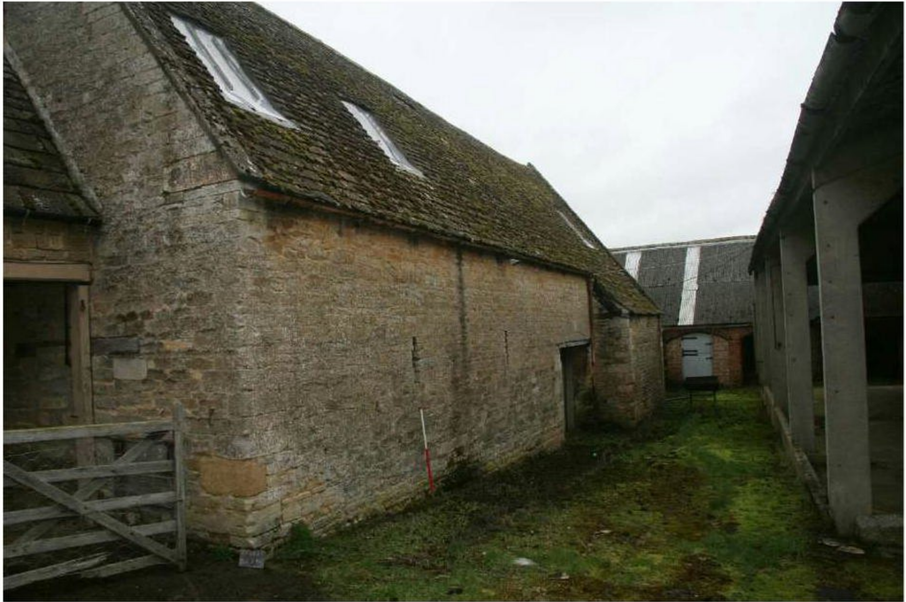
Plate 15: Building D, elevation 3, looking northeast
