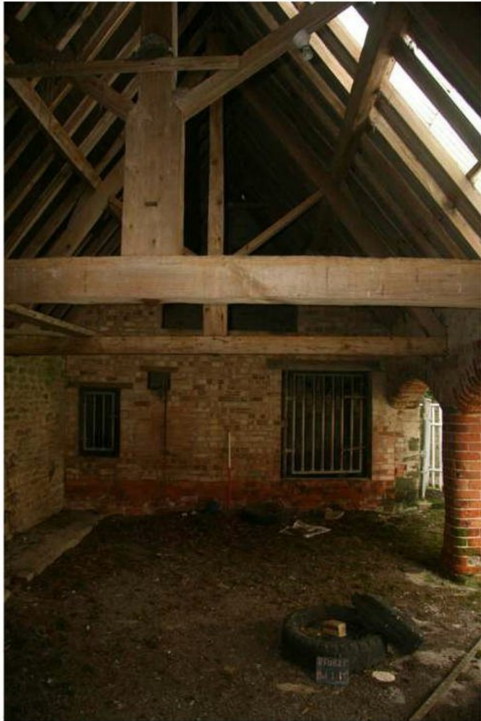
Plate 5: Building A middle room, looking south
