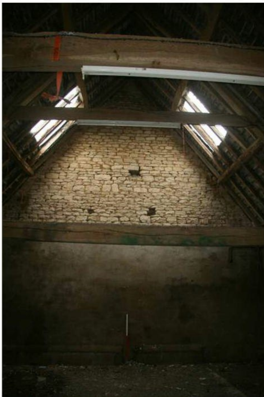
Plate 18: Building D, looking northeast
