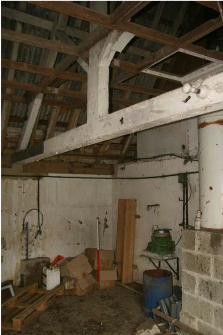
Plate 29: Building F, eastern room, looking southwest
