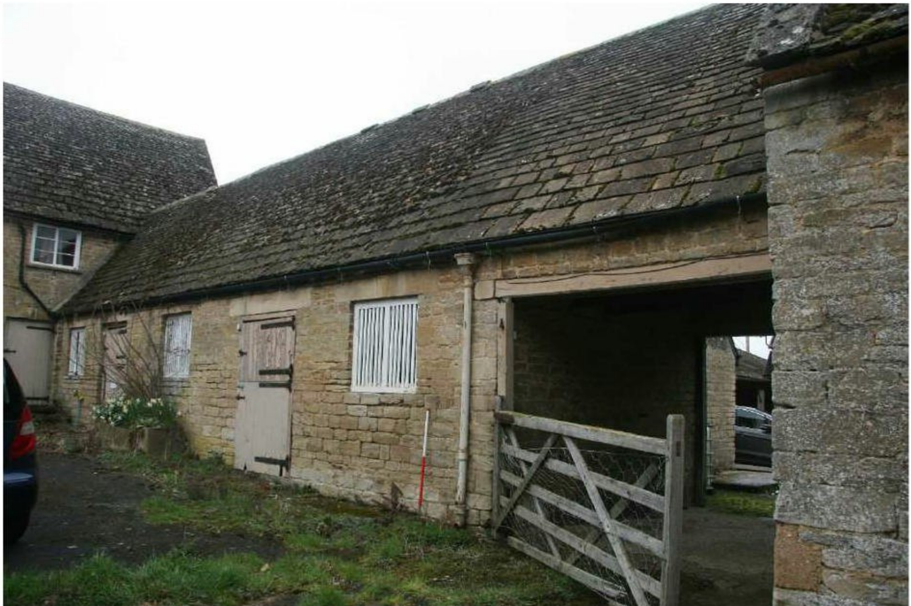
Plate 22: Building E, elevation 3, looking northwest.
