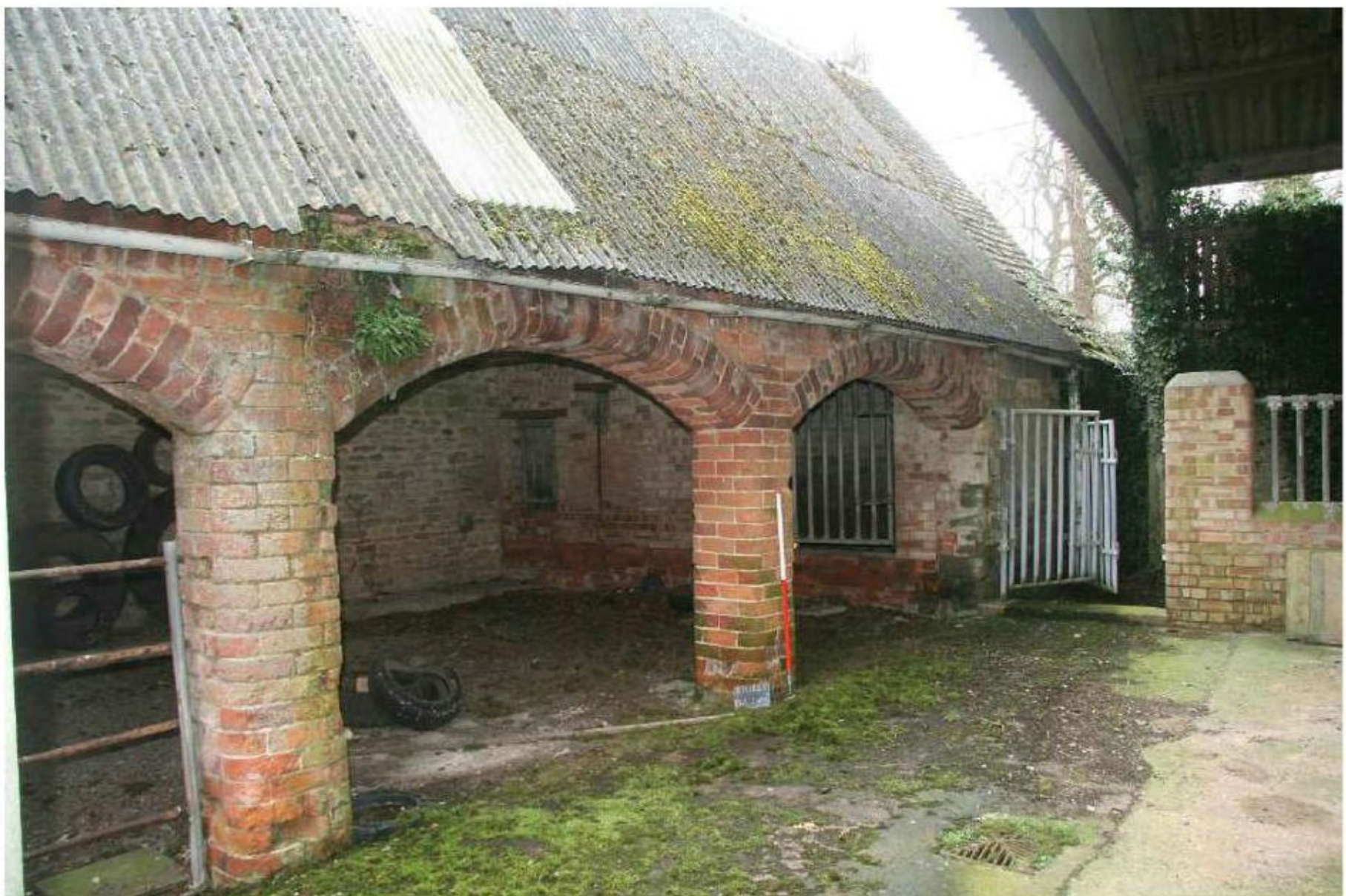
Plate 2: Building A, looking Southeast
