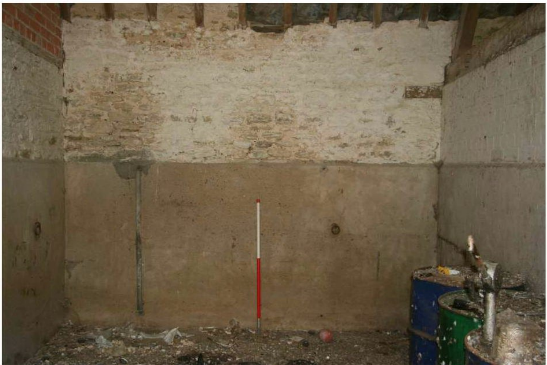
Plate 6: Building A, northern room, looking east
