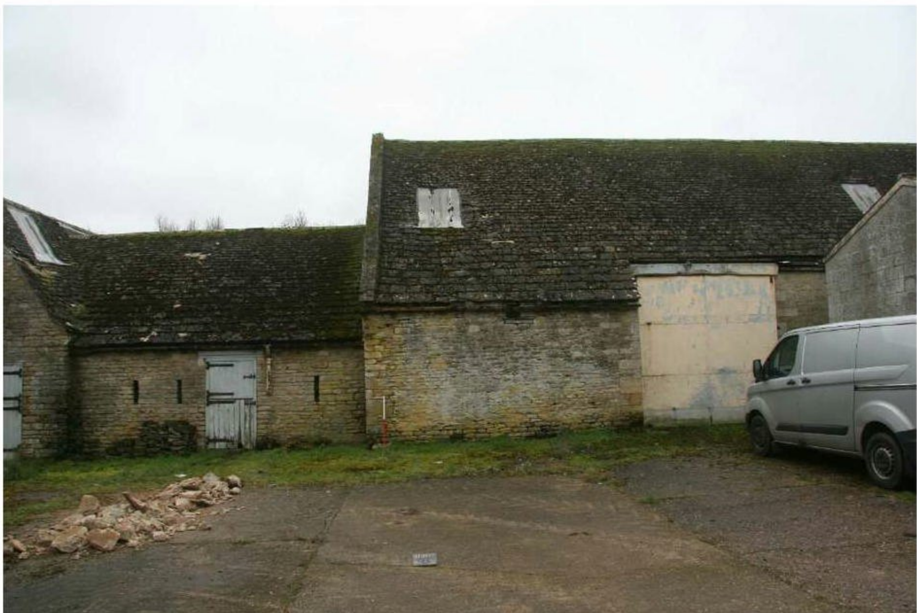
Plate 10: Building C and D elevation 4, looking south.
