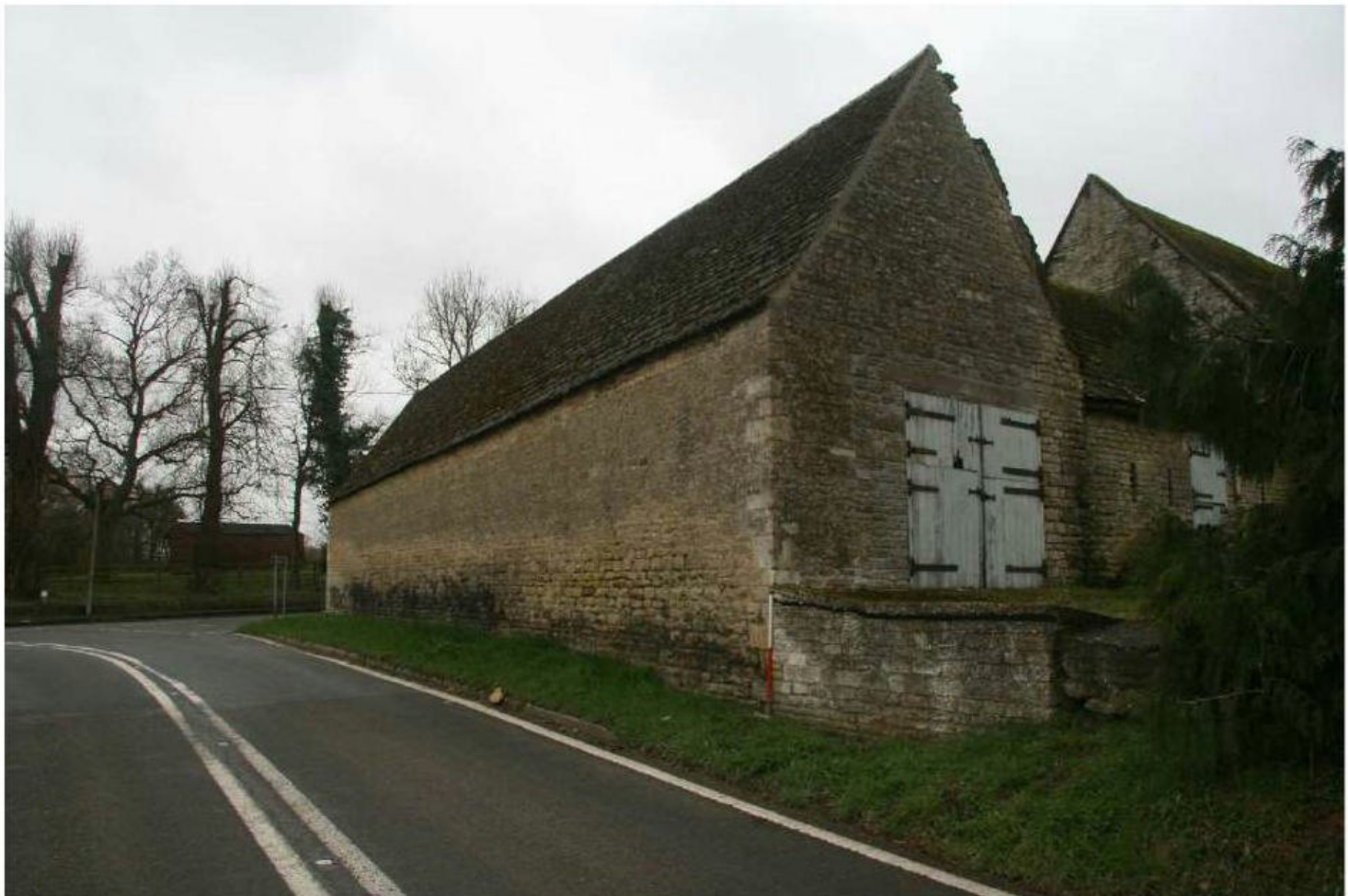
Plate 8: Building A and B elevation 2, looking northeast
