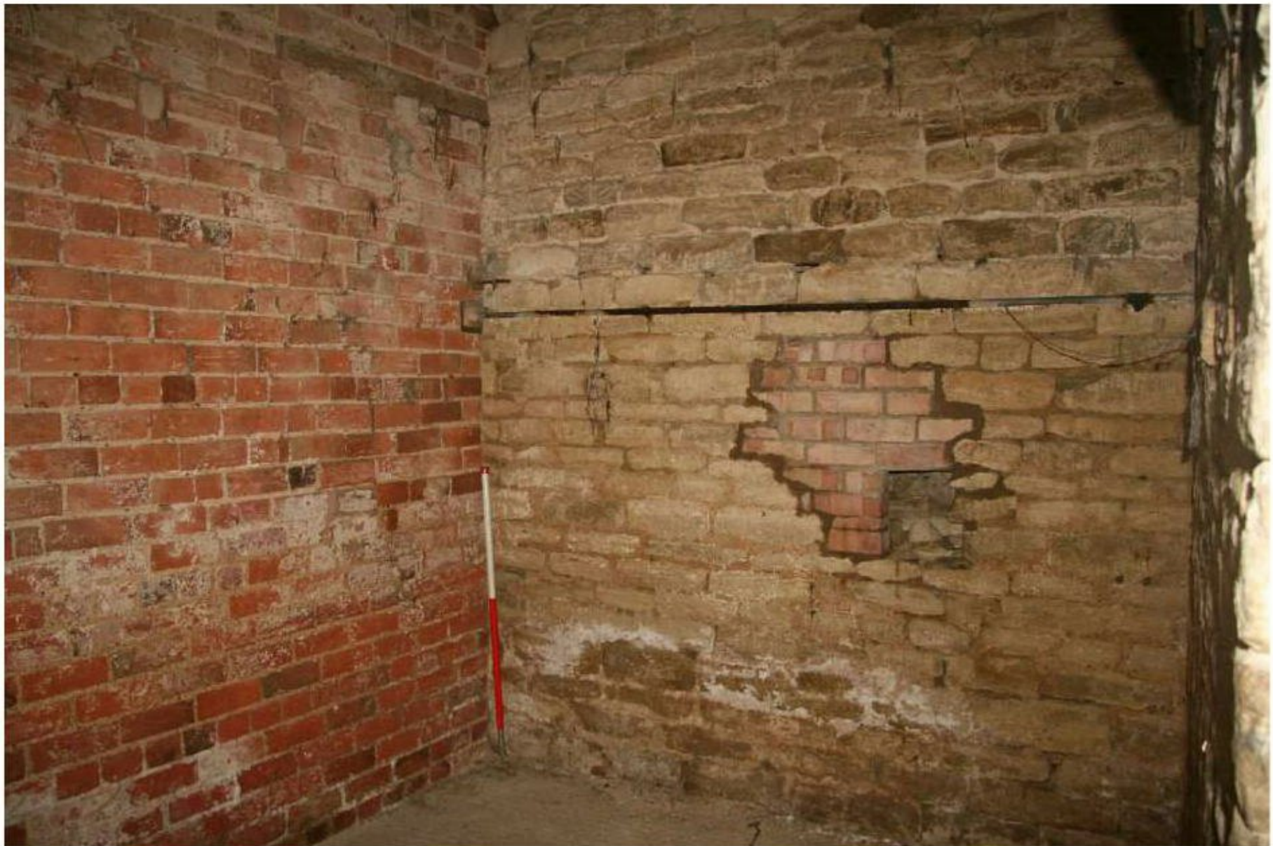
Plate 24: Building E, middle room, looking northwest.
