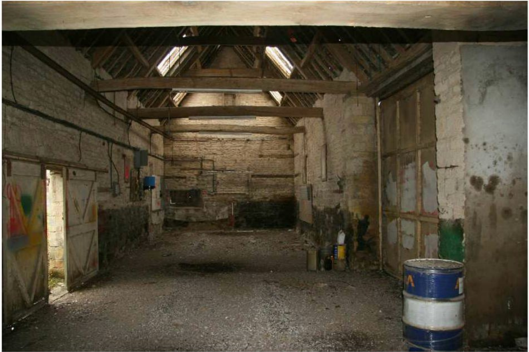
Plate 17: Building D, looking southwest
