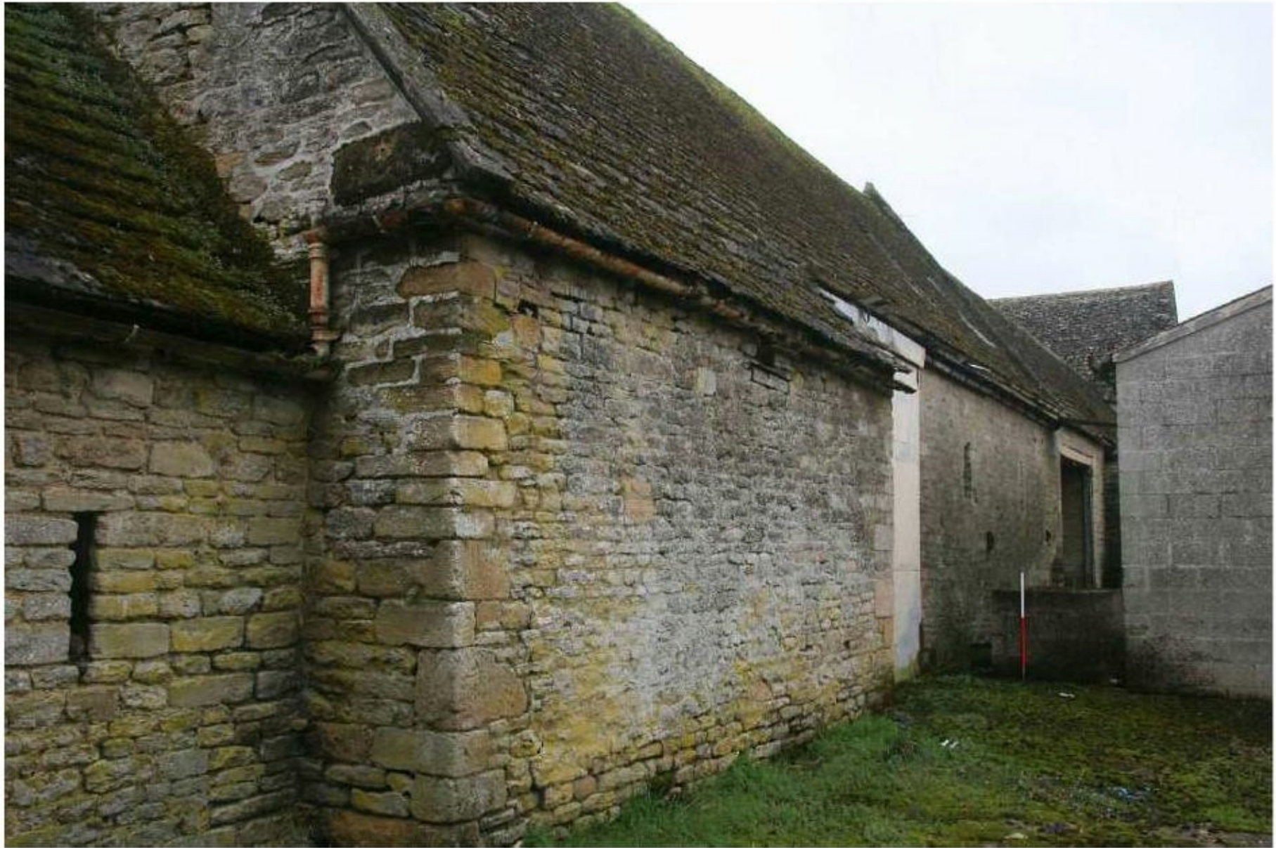
Plate 13: Building D, elevation 4, looking southwest.
