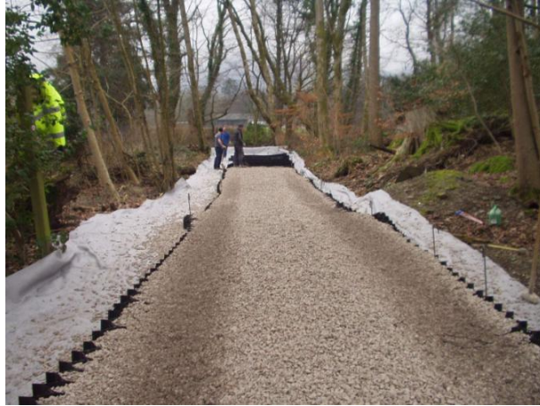
Photograph no.2: Aggregate fill
