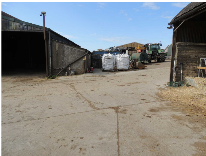
Photo 15: The farmstead. Note concrete hardstanding
