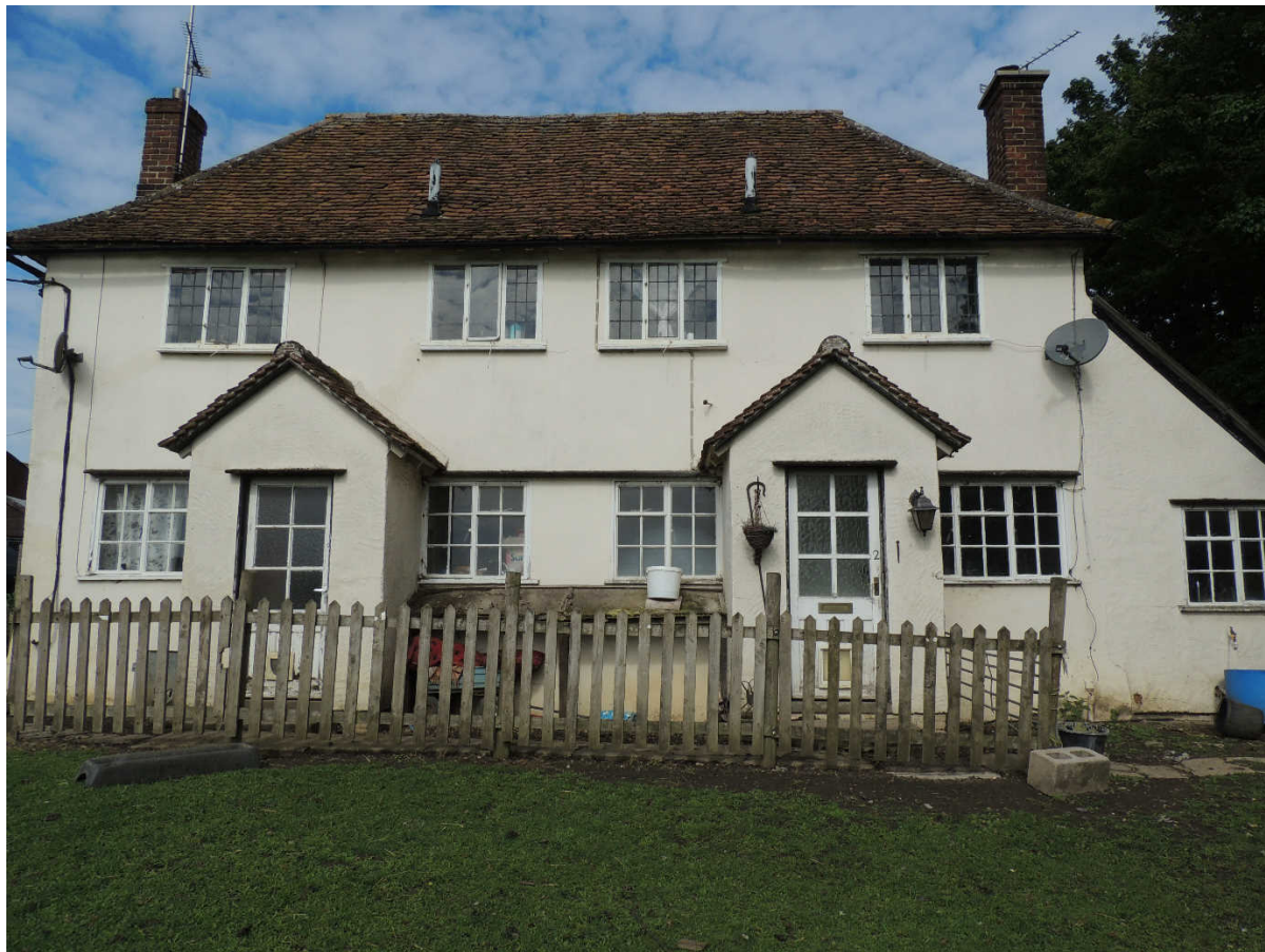
Photo 1: Front (eastern) elevation. The proposal is to demolish and replace the dwelling
