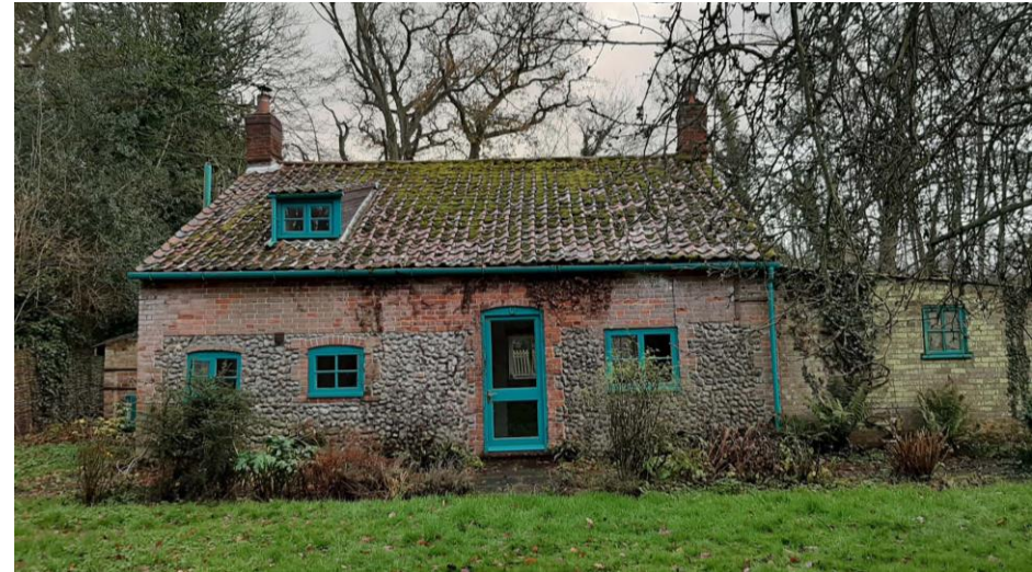
Photograph –Rear (North) Elevation
