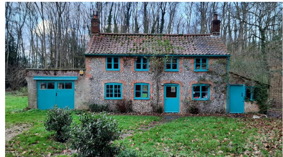
Photograph – Principal (South) Elevation
