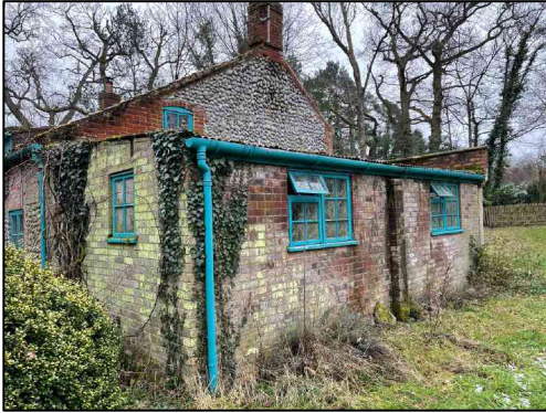
Figure 12 – View of the western gable
