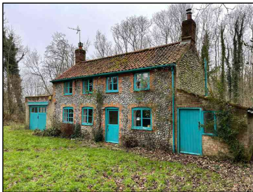
Figure 10 – View of the property from the south
