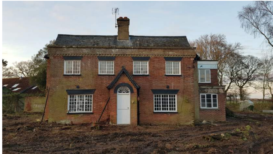
Photo of the South-East facade and porch structure that is to be retained
