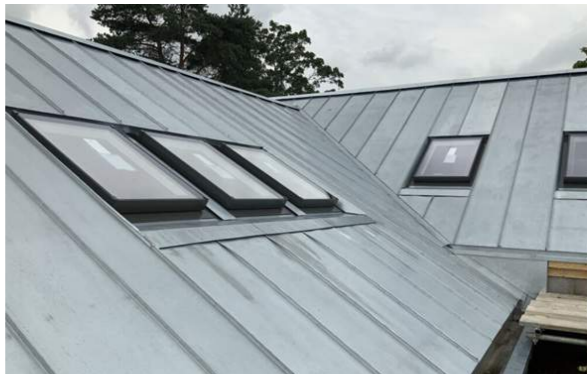
The new pitched roof slopes will consist of standing seam zinc (dark grey or naturally weathered in colour) zinc is a historic cladding material that requires little or no maintenance. This material appears quite agricultural when installed, minimal detailing and recessed gutters will result in a slightly contemporary take on this traditional aesthetic.
