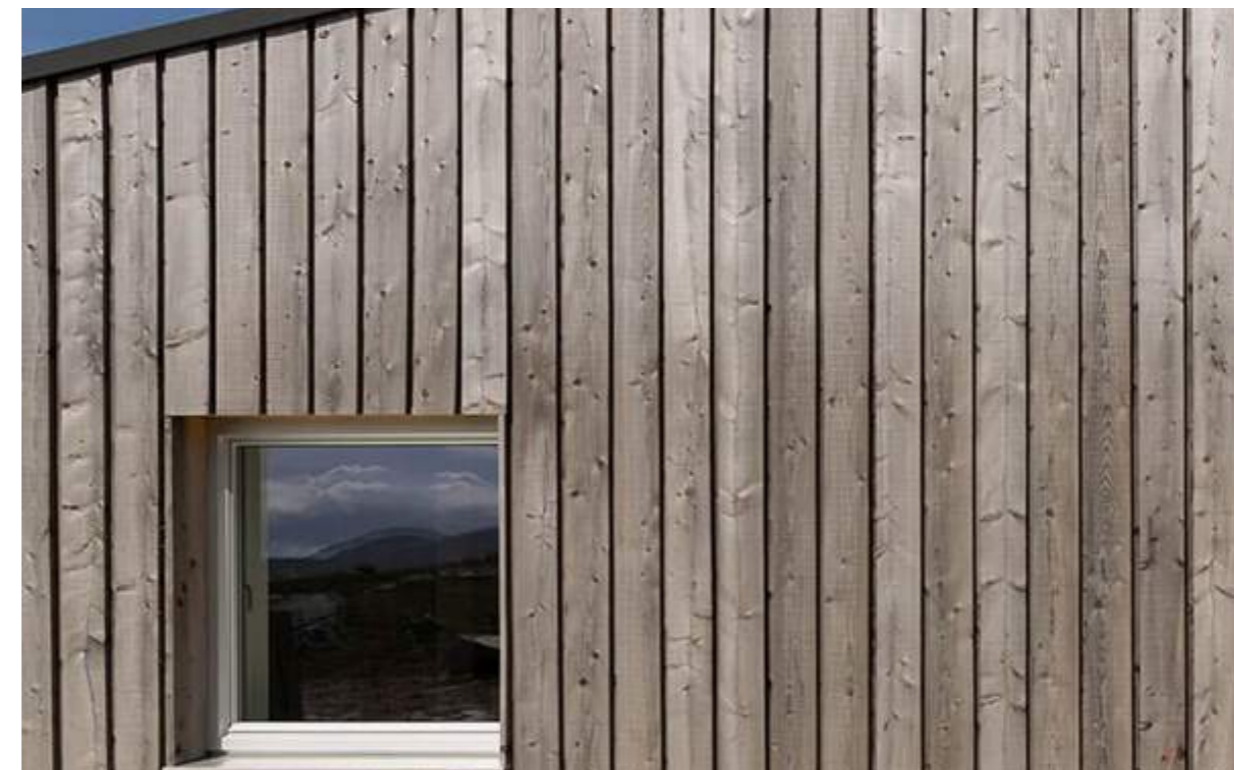
The external walls of both the East and West elements will be clad using Siberian Larch. This will be installed as vertical boards and be left to weather in its natural state. Siberian Larch achieves a natural patina extremely quickly (1 season) and is superior in this respect to alternative materials such as Cedar. No treatment or maintenance of this product is required as this slow growing timber contains natural preservatives.
