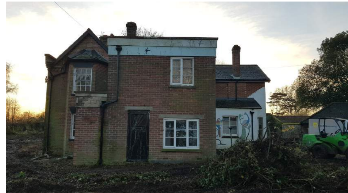
20th Century flat roof additions
