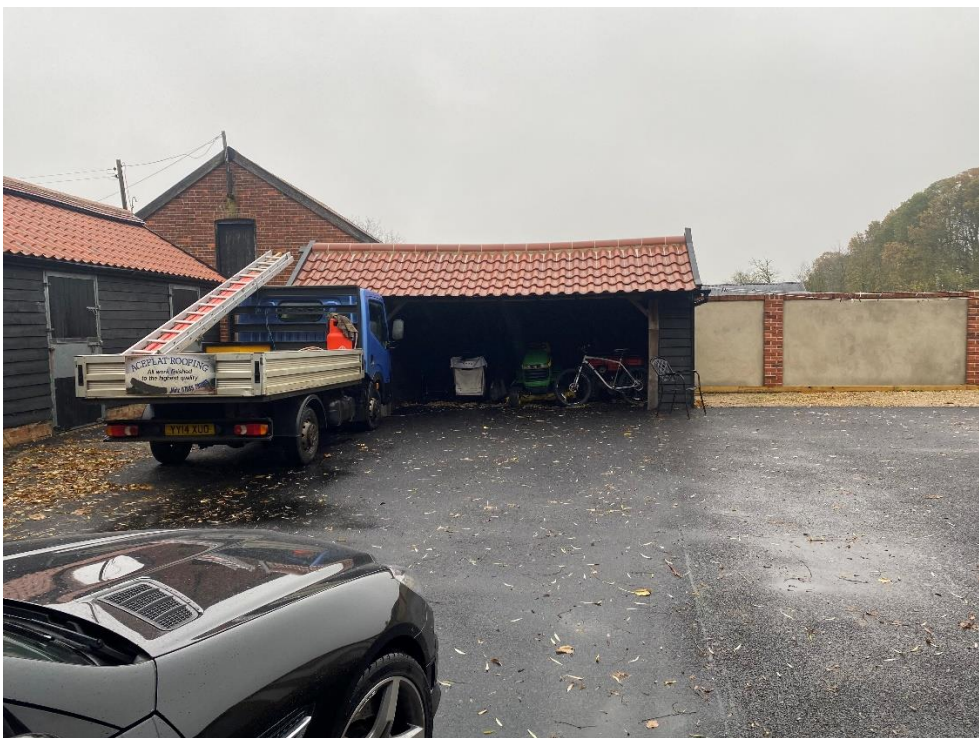
Photo 2. View looking east towards the position where the new building is to be erected.
