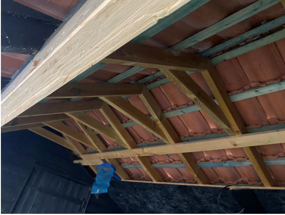
Photo 3. Interior roof of building to be demolished.
