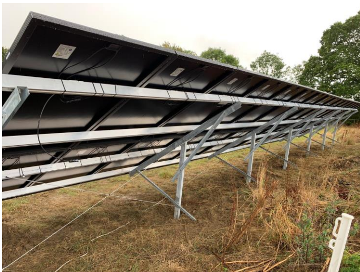
Examples from previous ground mount installation
