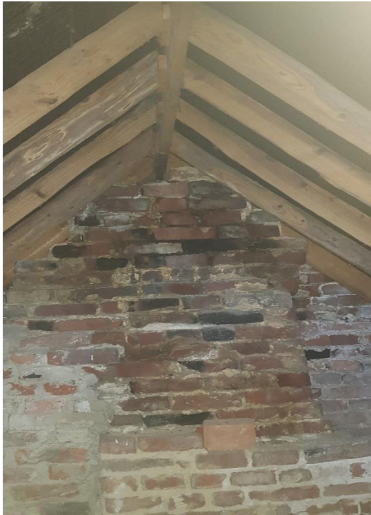
Picture 5: Showing the internal roof space
