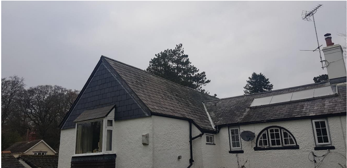
Picture 2: Showing the rear, southern elevation.
