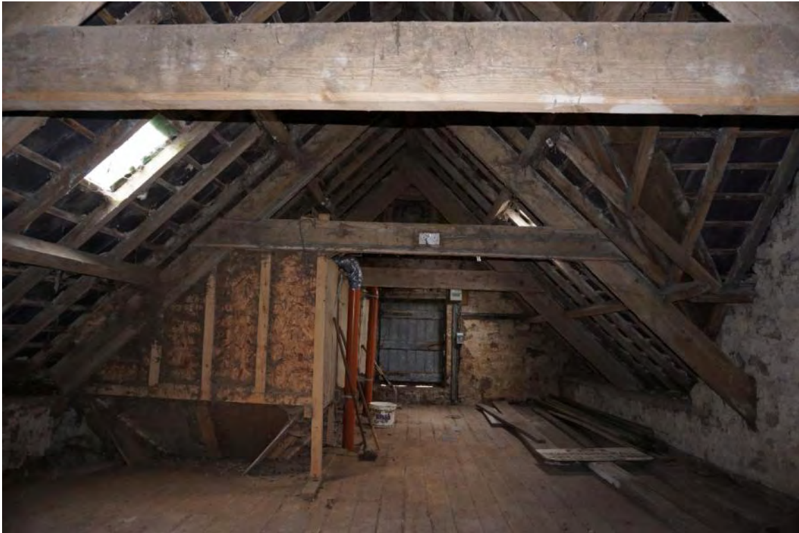
PHOTO 12 – Main Hayloft over stables – 3 trusses, top of hoppers to left.
