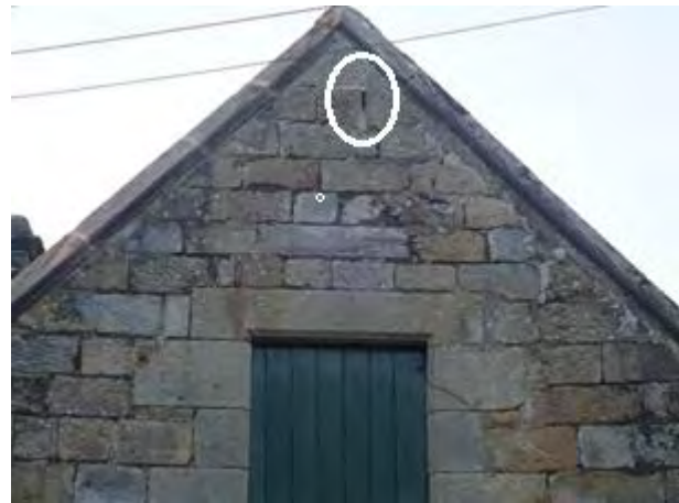
South Gable crevice to be retained
