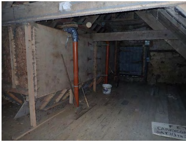
Interior of the north loft
