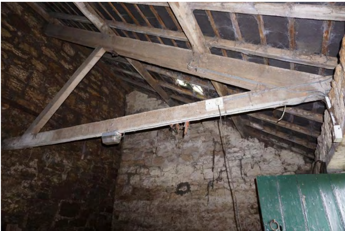
PHOTO 13 – Triangular trusses to roof of stables on north side
