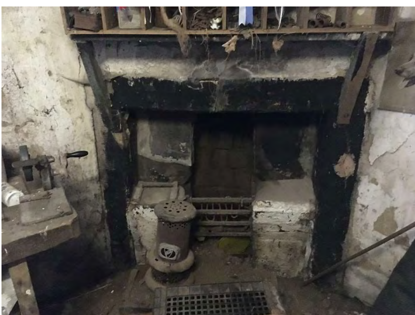
Photo 12 Internal view of former Groom's Cottage fireplace.
