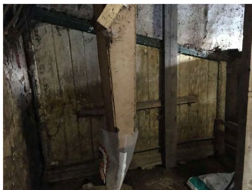
Photo 11 Internal view of former stable east end panel behind 1960s feed hopper.
