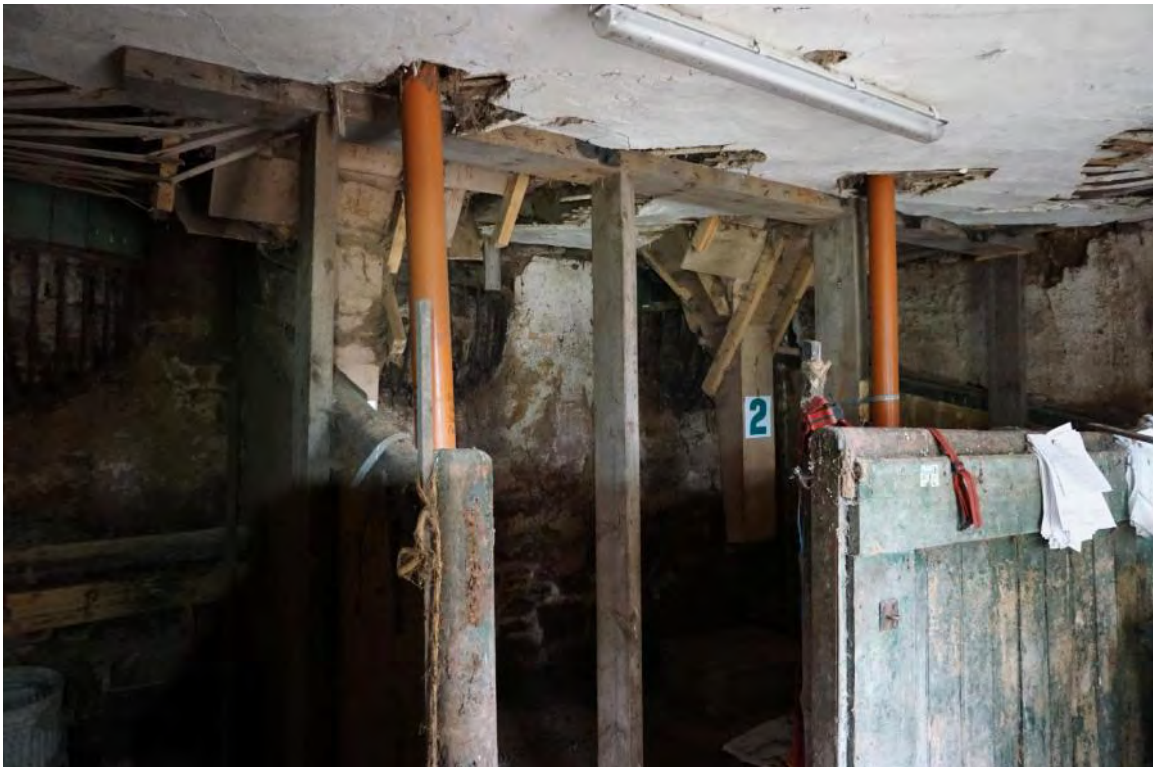
PHOTO 9 – Timber Props to Joists in Stables – joists cut to accommodate hoppers
