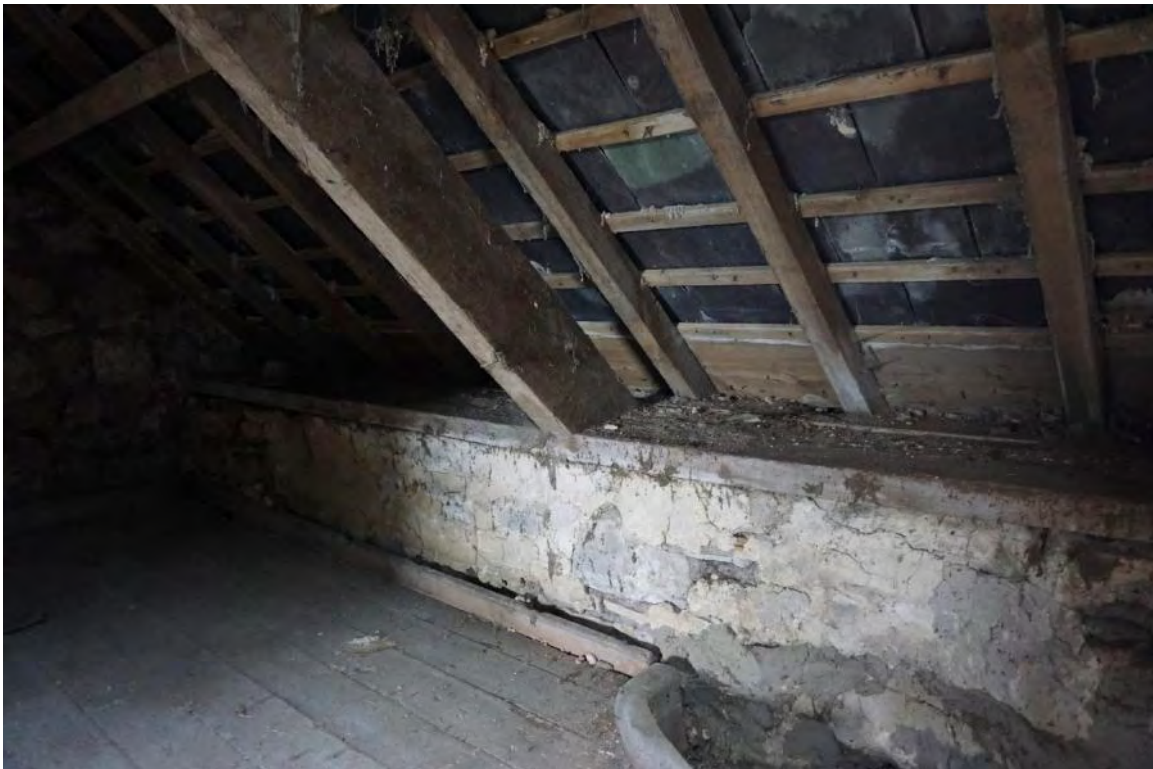
PHOTO 11 – Truss end detail – timber wall plates
