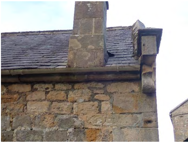
West eaves, showing raised slates
