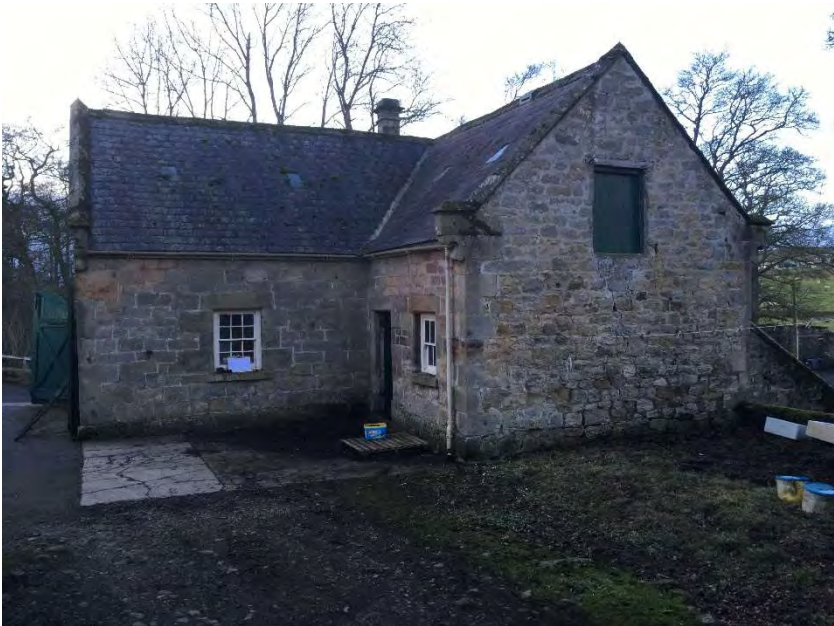
Photo 9 Coach House from east.
