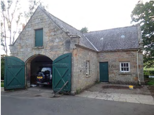
The coach house from the south
