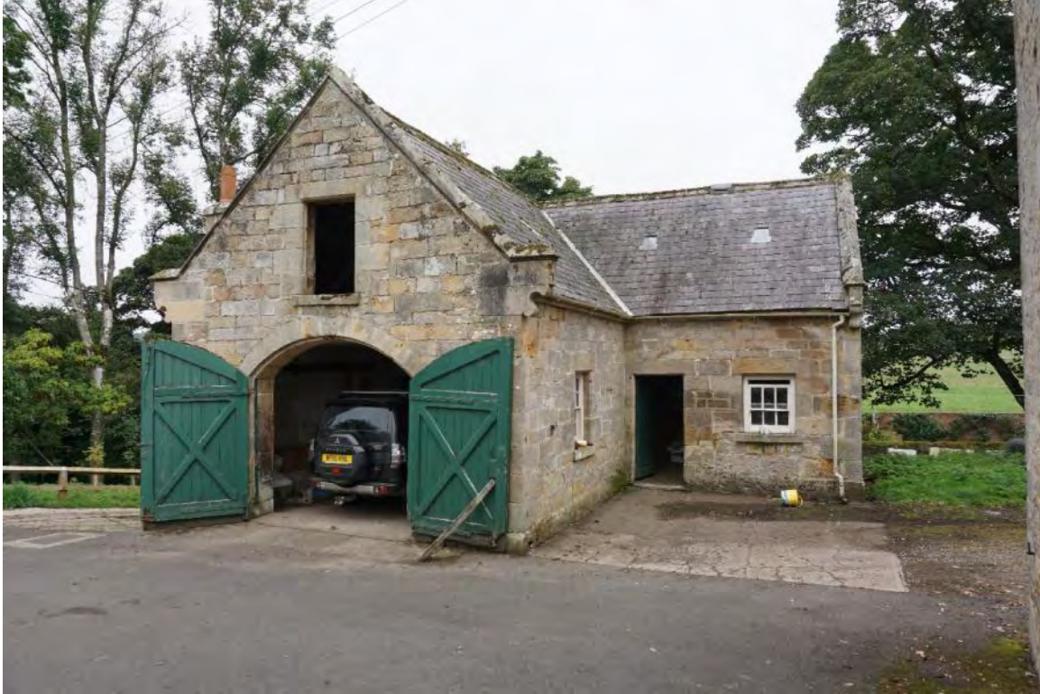
PHOTO 1 – Front Elevation (south)
