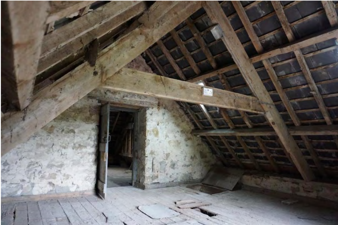
PHOTO 10 – Truss above coach house
