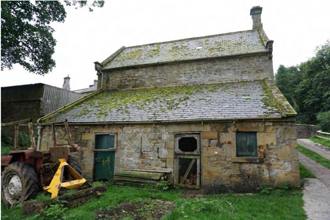
PHOTO 3 – Rear Elevation (north)
