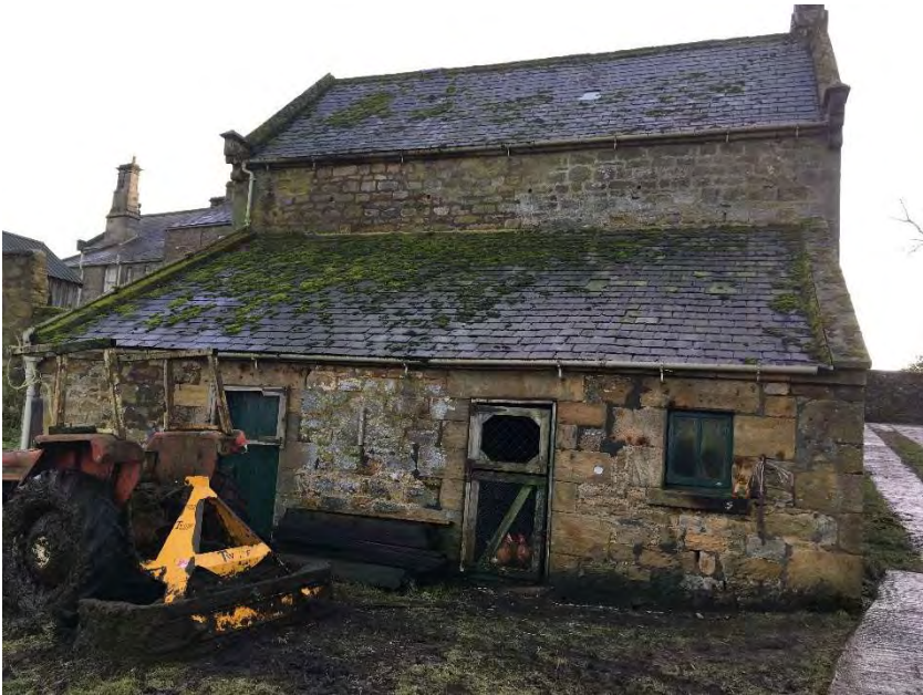
Photo 7 Coach House from north with lean-to in foreground and Carrycoats Hall behind.
