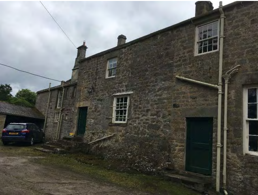
Photo 4 Carrycoats Hall north wing from northwest.
