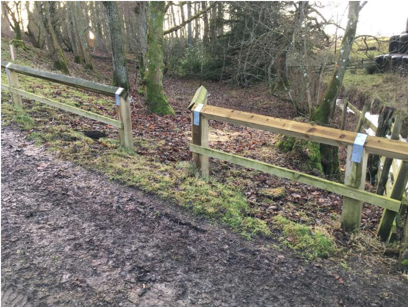
Photo 20 Existing birds-mouth fencing to west.
