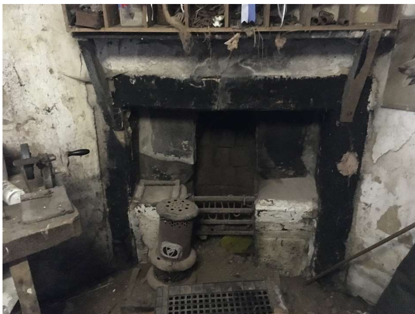
Photo 12 Internal view of former Groom's Cottage fireplace.
