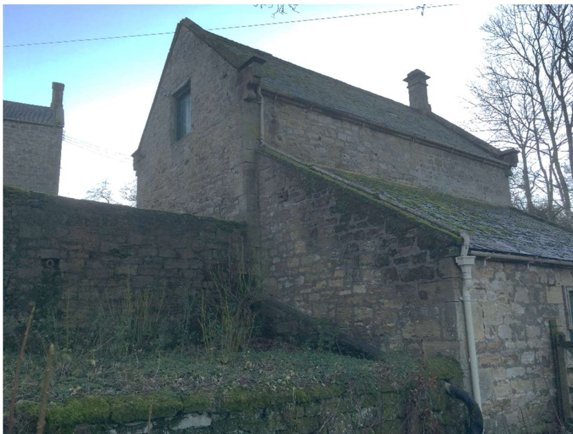
Photo 8 Coach House from northeast.
