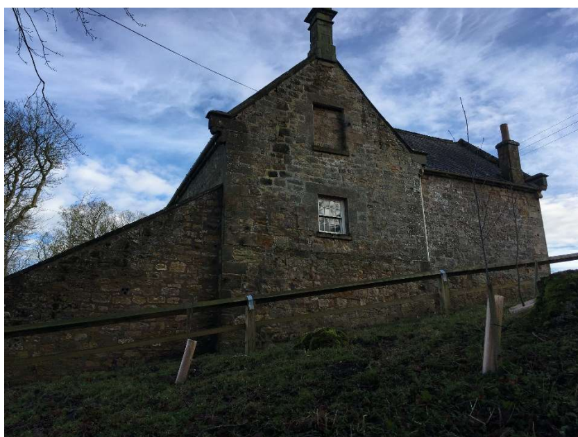
Photo 6 Coach House from west.
