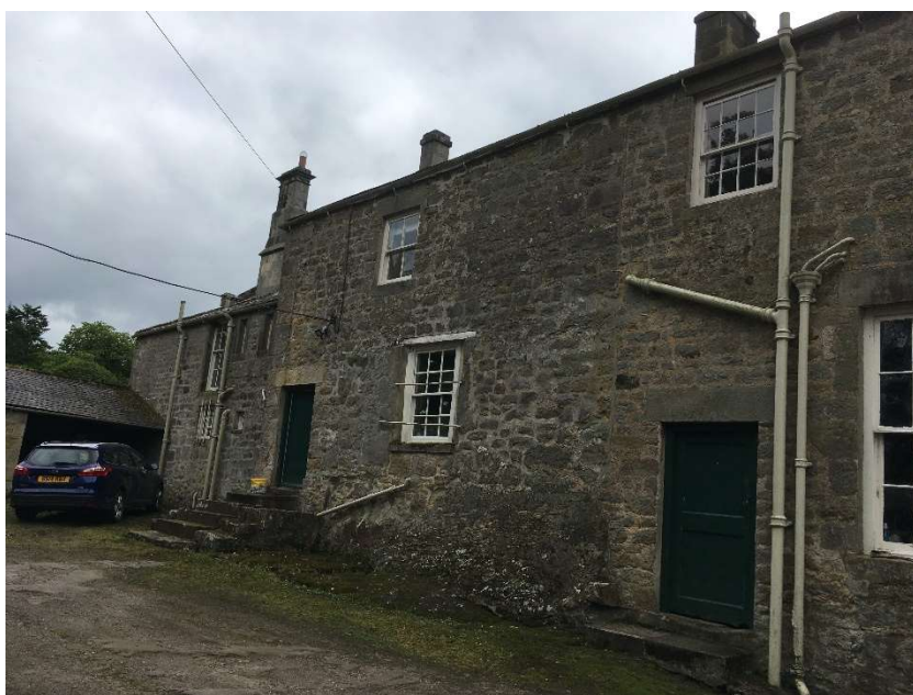
Photo 4 Carrycoats Hall north wing from northwest.
