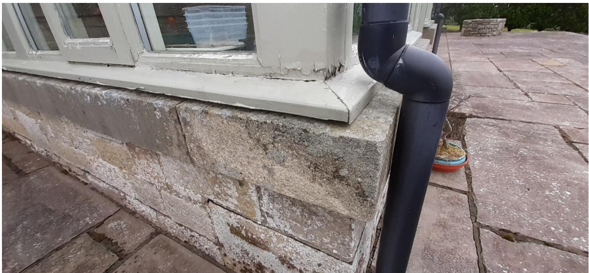
Fig 7: Close up of stone plinth and window cill detail
