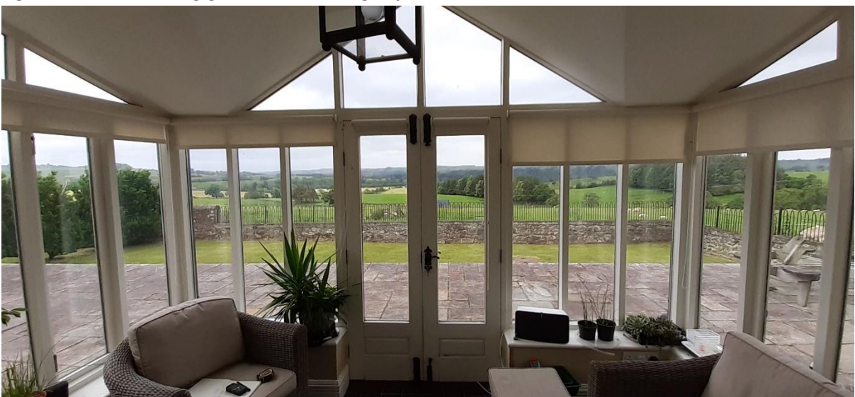
Fig 4: Inside the existing glass house looking south at the view over North Tyne valley
