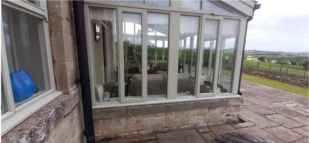
Fig 6: West elevation of glass house showing low stone wall and vertical fenestration
