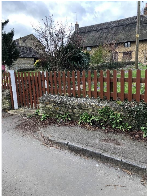
View of existing garden wall
