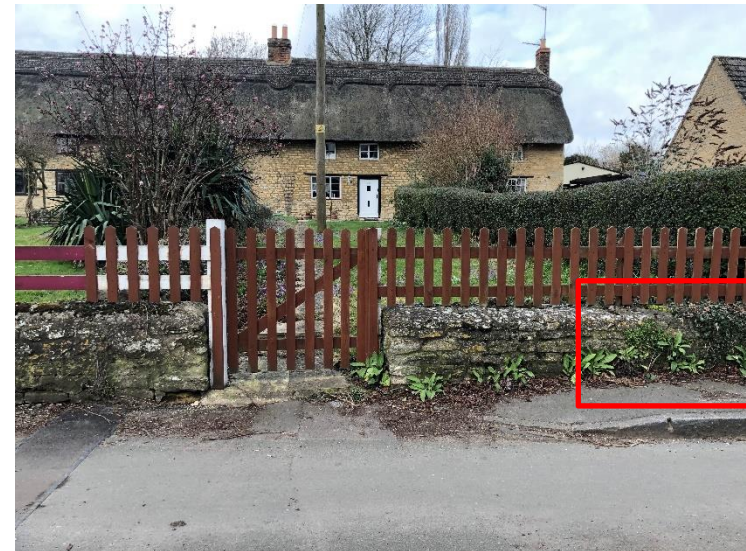
View to existing drop kerb and opening within wall
