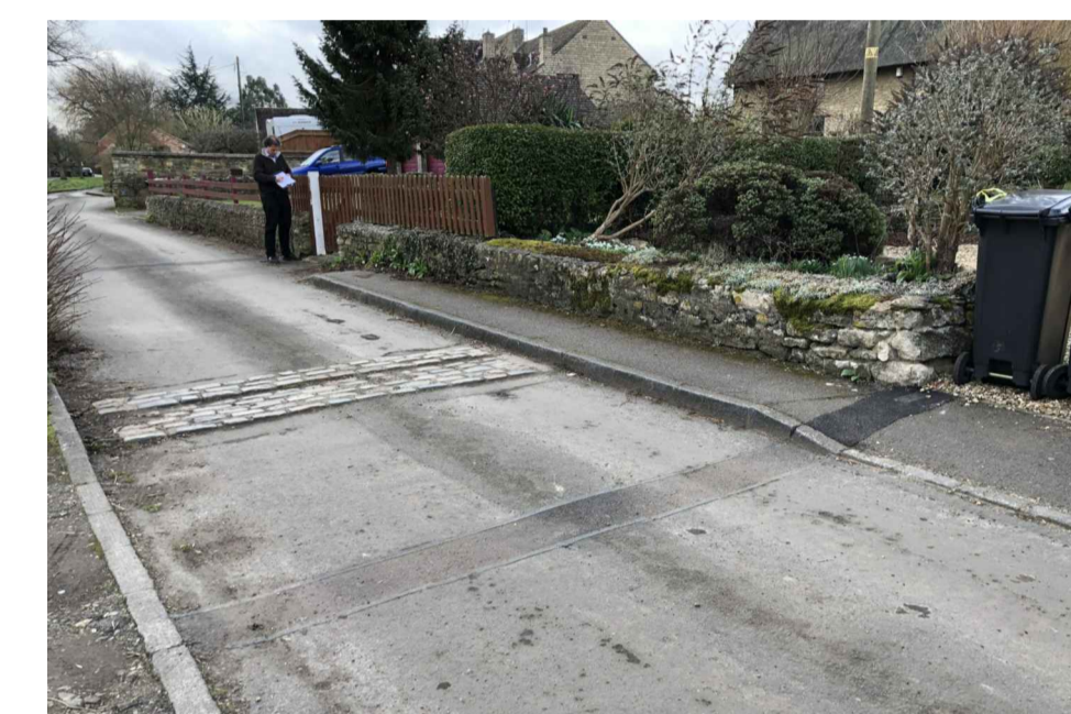
SURVEY PHOTOGRAPH 1 (P1)
