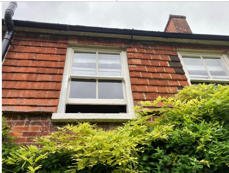
Photograph 3: Hanging tiles bonded to wall on the southern side of the building.
