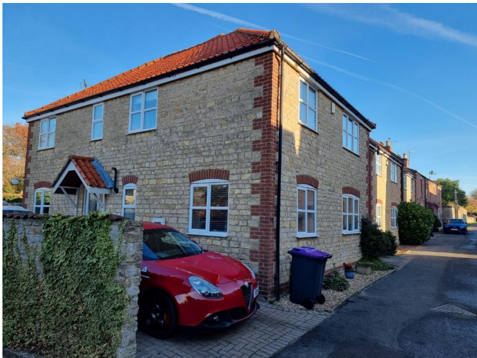
View of property from Far Lane
