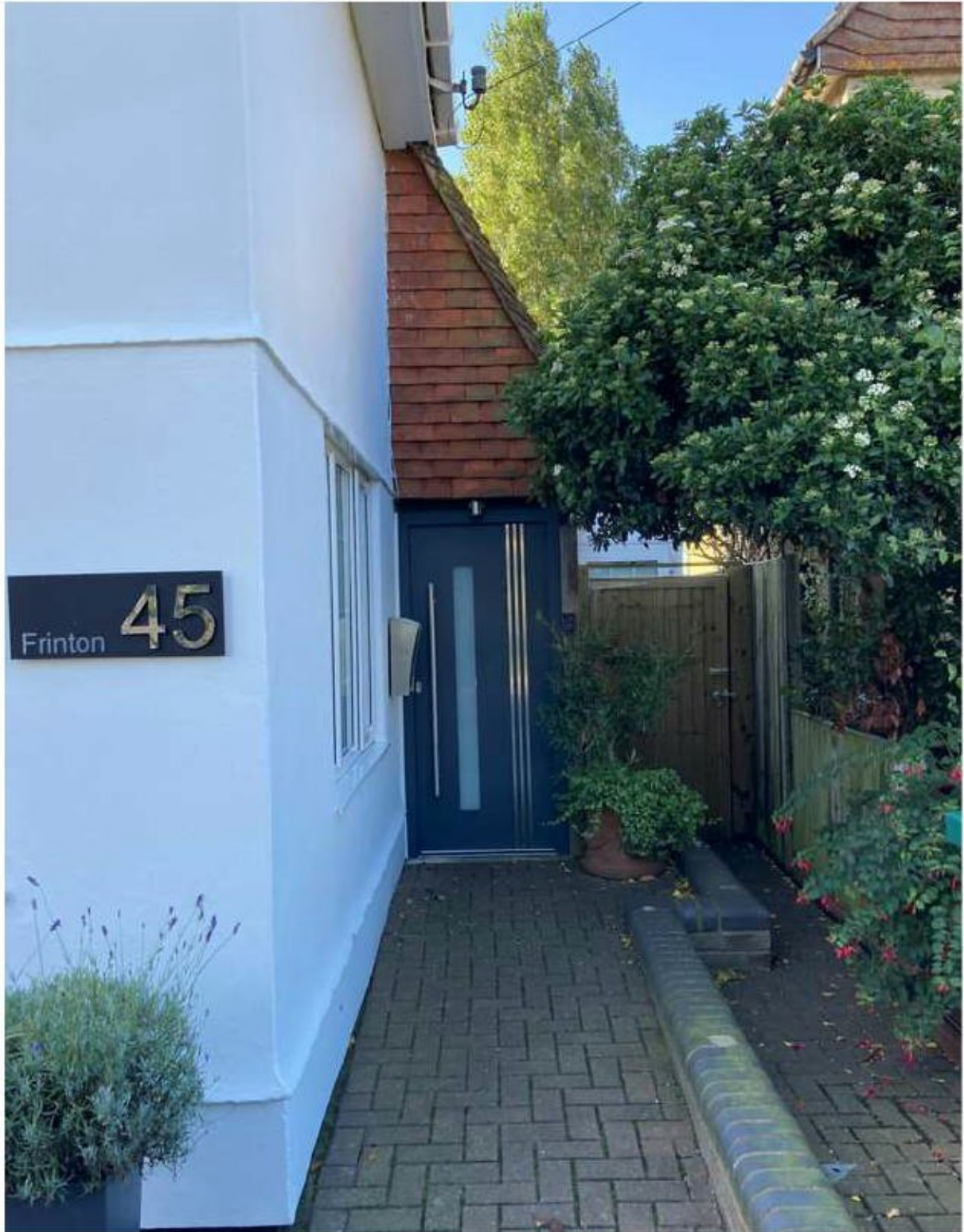
Fig. 3 – Front view showing front door and existing conservatory structure behind gate to RHS.
