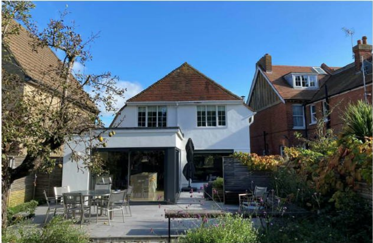
Fig. 6 – Rear view of main house – note extension & #43 to RHS
