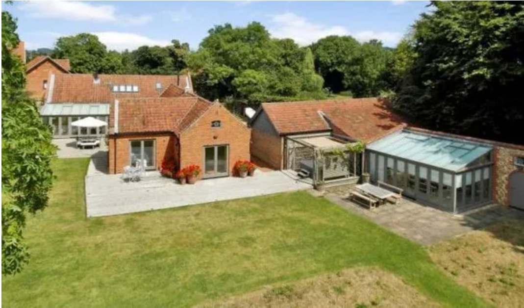
Existing view showing conservatory to right replaced similar design with conservatory at back subject of change to orangery style to reduce solar gain and improve thermal efficiency.
