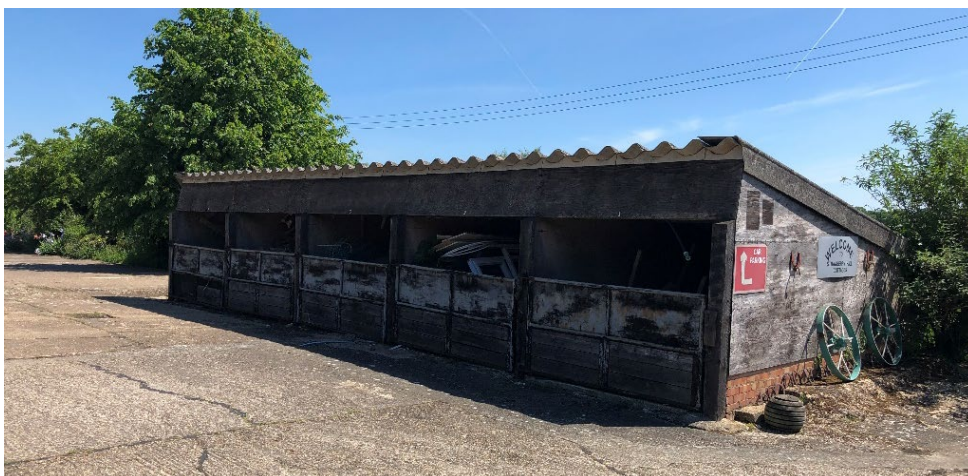
3. Garage to be demolished
