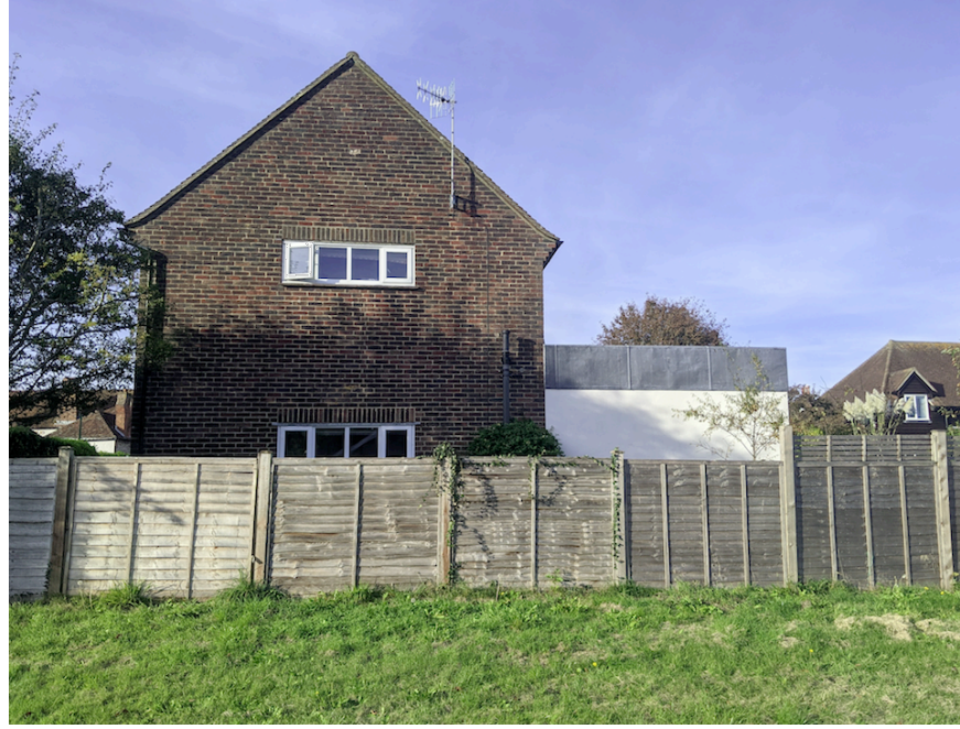
Photograph (2) Side (South) Elevation
