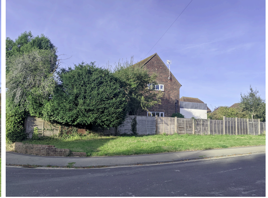
Photograph (3) Side (South) Elevation
