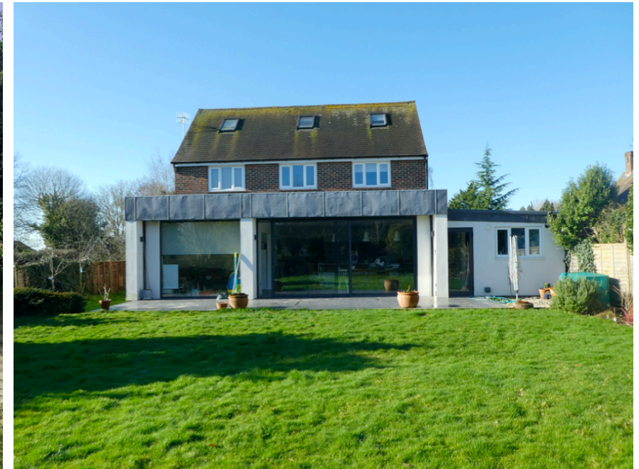
Photograph (6) Rear (East) Elevation
