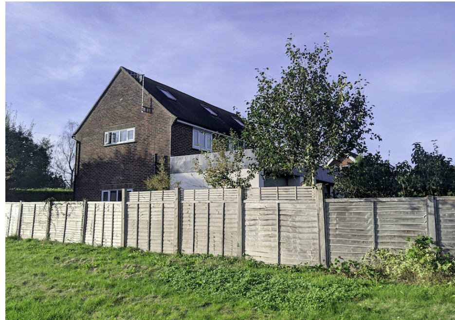
Photograph (4) Side / Rear (South / East) Elevation
