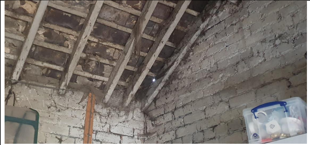
B1 internal roof structure
