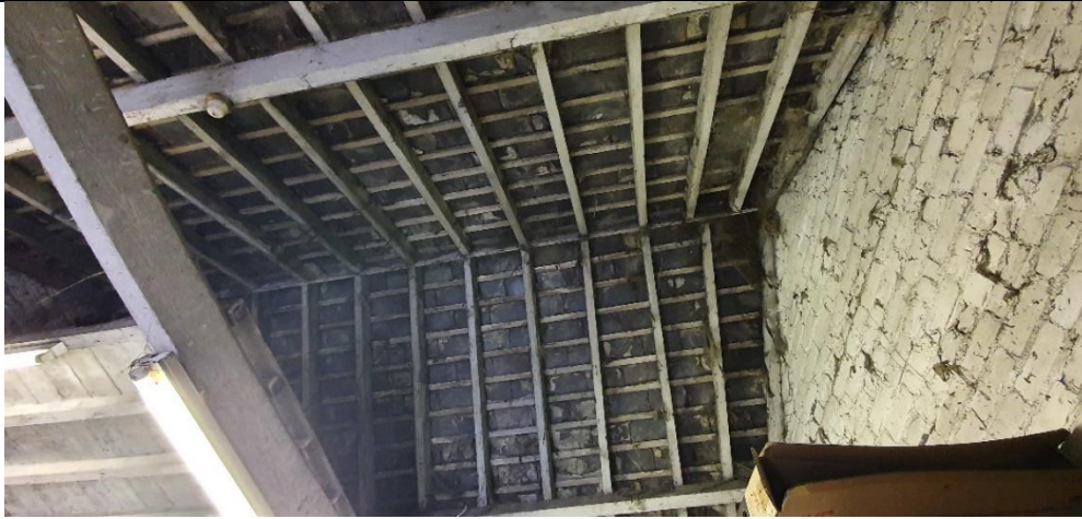
B1 internal roof structure
