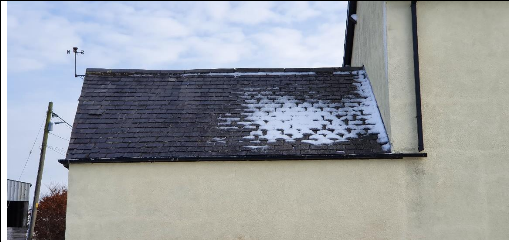
B1 western elevation roof (pictured above).
