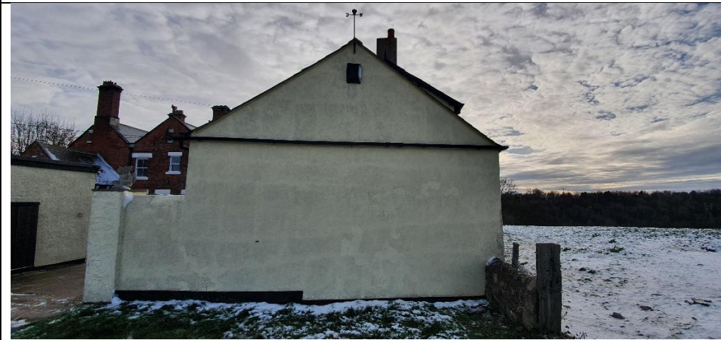
B1 northern elevation gable end (pictured above).
