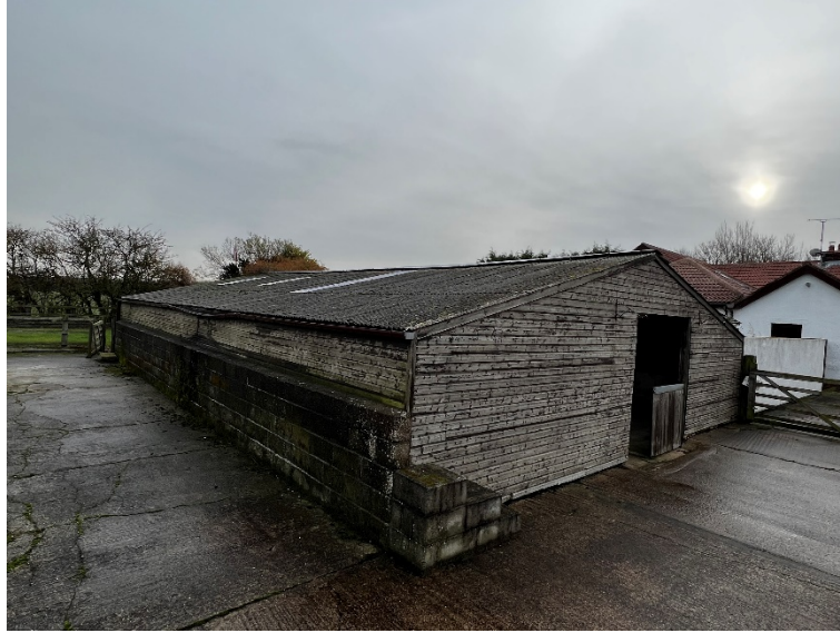
Plate 1 – north elevation and west gable.
