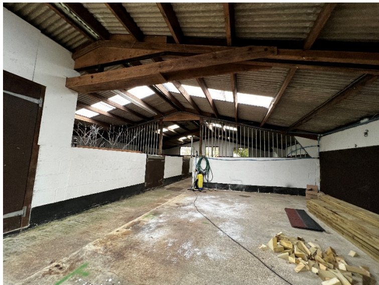
Plate 3 – internal roof void
