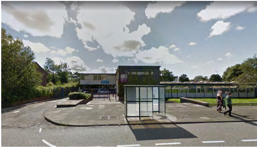
4.0 Fig. 1 View from High Street, showing the existing bus stop and Co-Operative offices currently on the site
