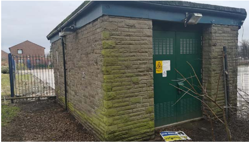
4.0 Fig. 5 Existing sub-station on site
