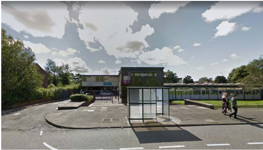
4.0 Fig. 1 View from High Street, showing the existing bus stop and previous Co-Operative offices on the site, which have since been demolished
