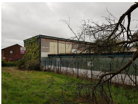
Photo 2 northern aspect of building, flat roof, timber barge board and boarded windows.
