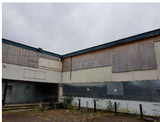
Photo 7: timber boarding on the north-eastern aspect.
