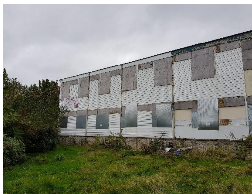
Photo 3: PVC cladding and timber boarding on southern aspect of the western section of the building.
