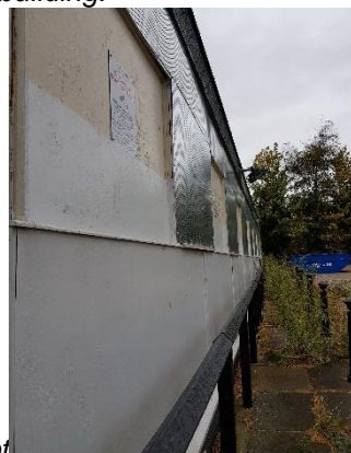
Photo 3: PVC cladding and timber boarding on southern aspect of the western section of the building.
