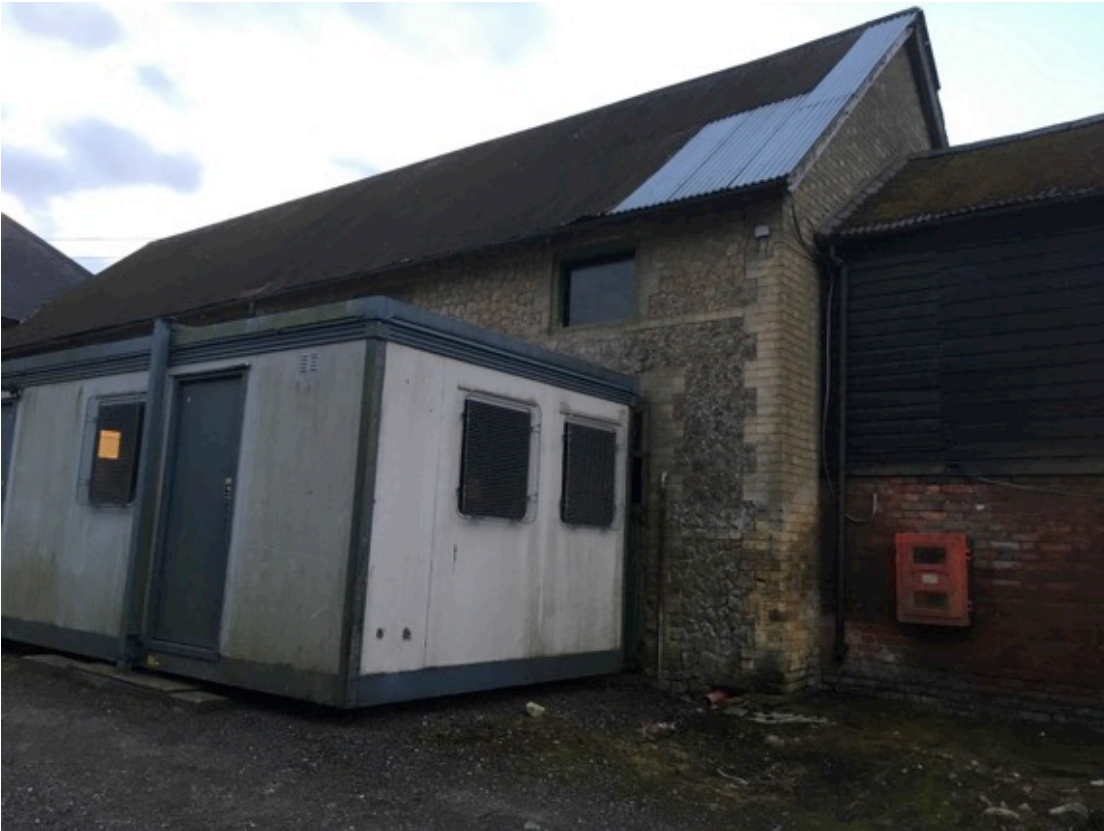
Photograph 9: Office block/middle (building 8)
