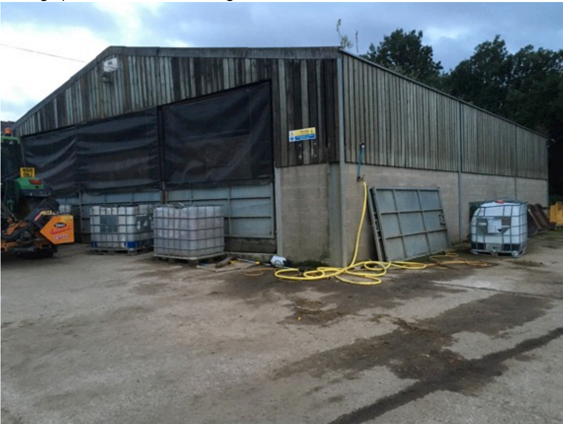
Photograph 14: Calf shed (building 12)
