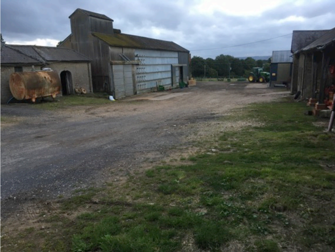
Photograph 1: View from the site entrance, looking west
