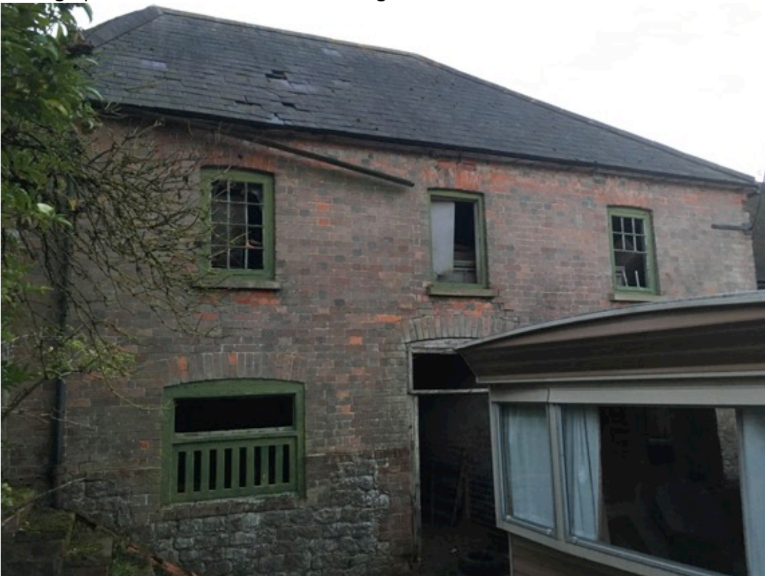
Photograph 10: Office block/rear (building 8)
