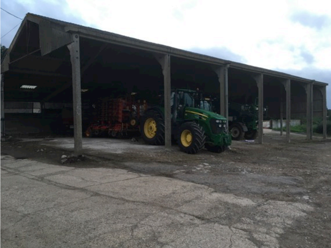
Photograph 12: Tractor shed (building 10)
