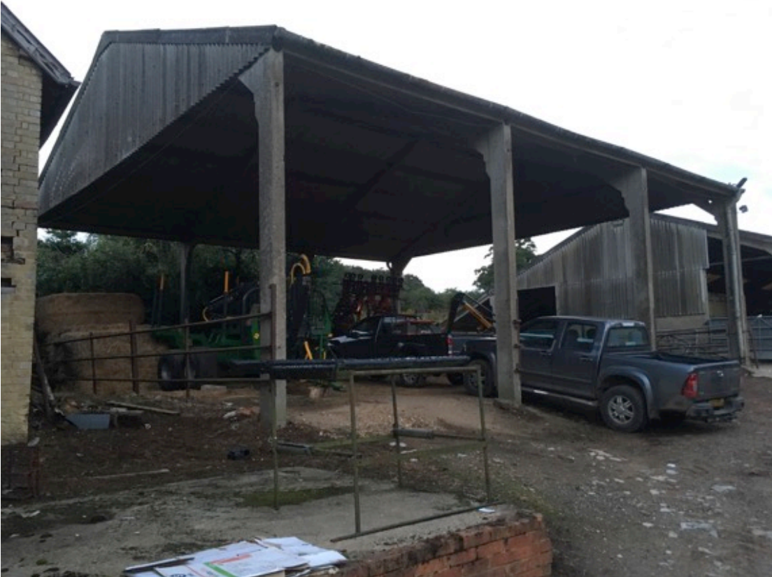
Photograph 11: Straw barn (building 9)
