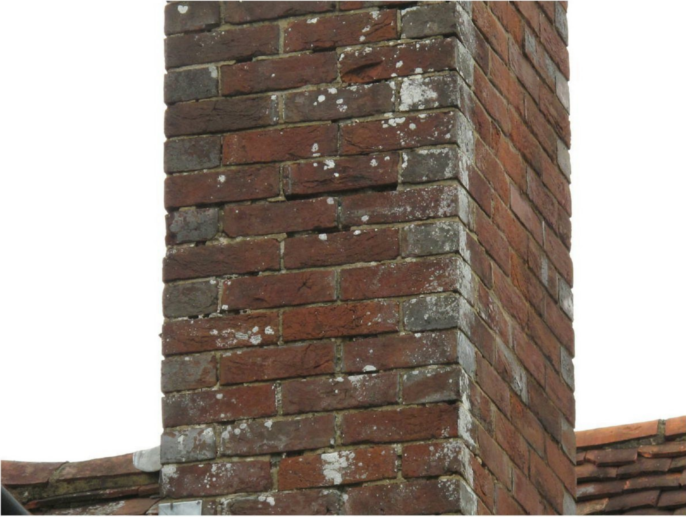
17. Detail of chimney
