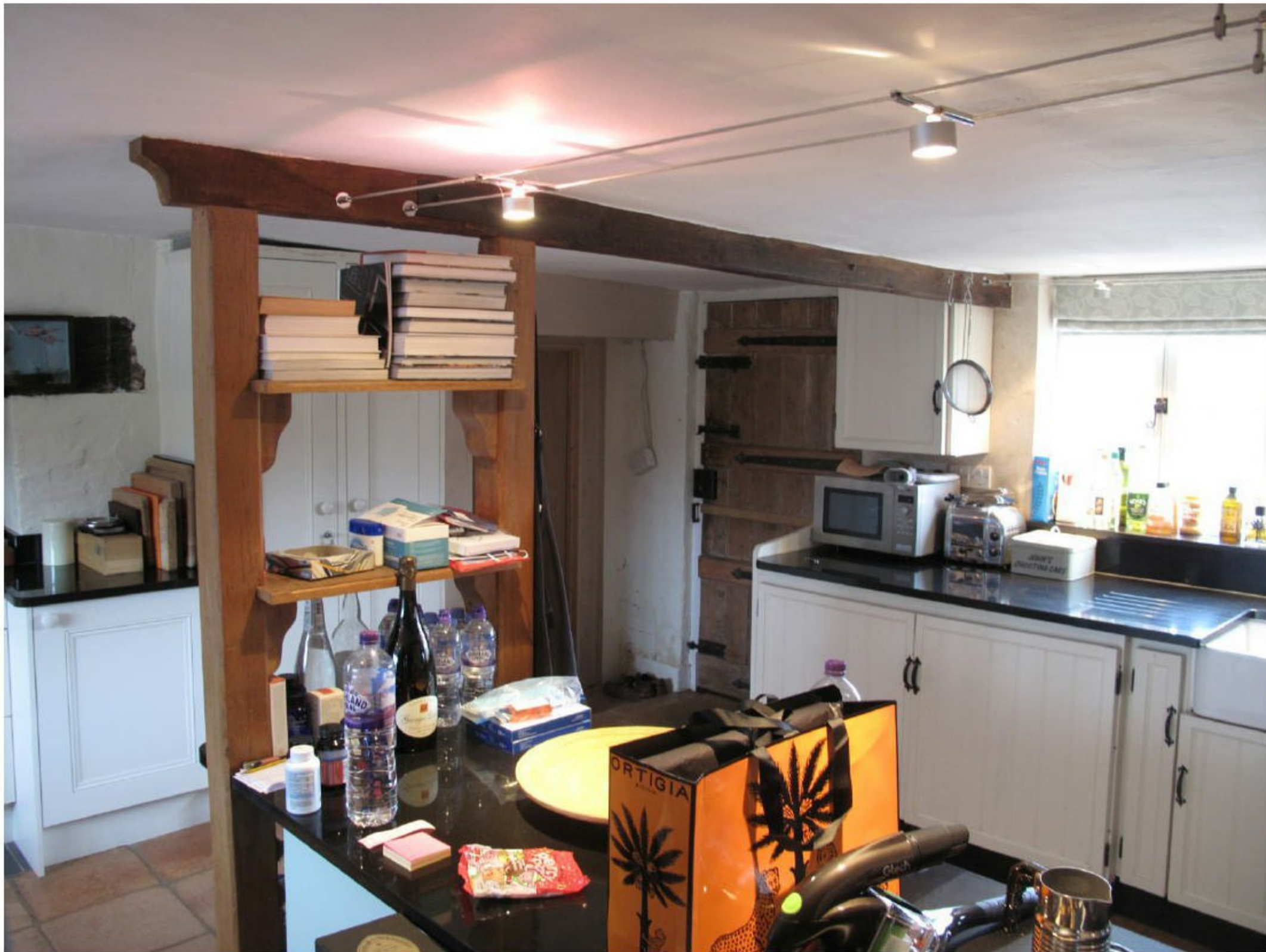
1. Investigate if posts and beam provide support to floor above
