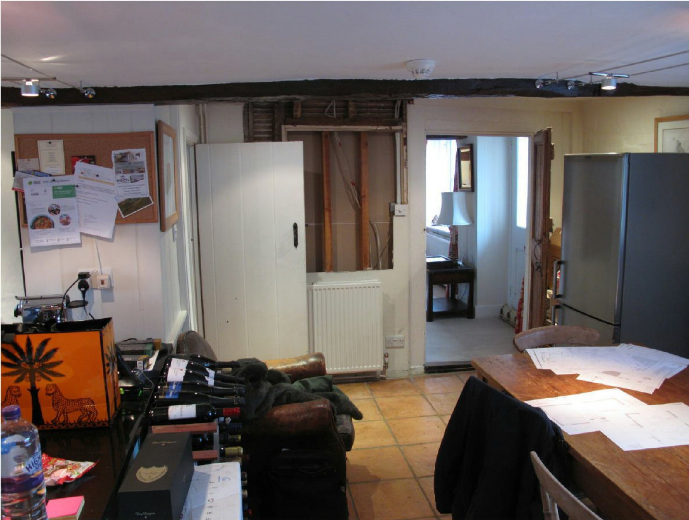
3. Stair enclosure and finishes to stud wall to be removed
