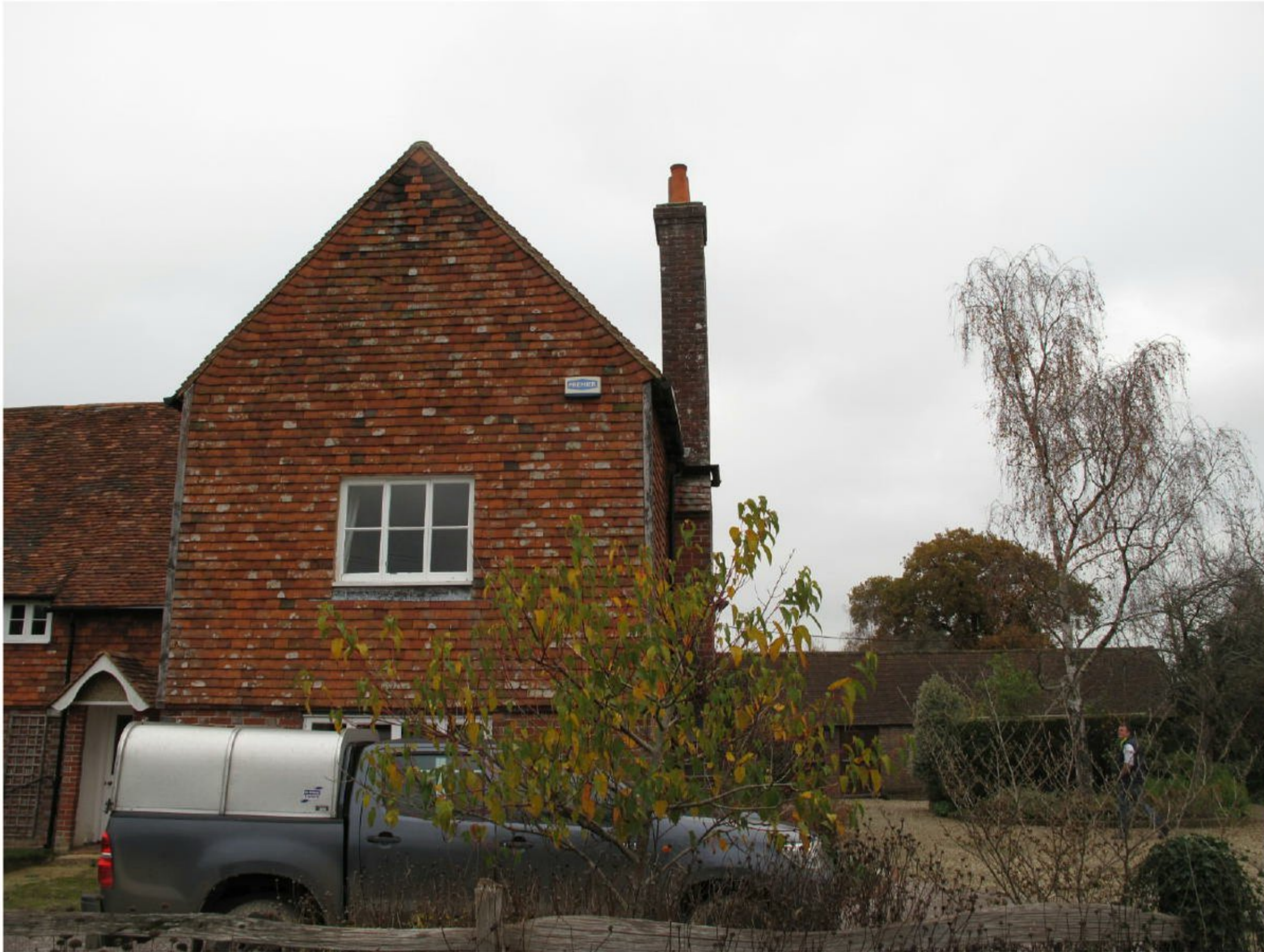
15. Chimney also leans towards the west
