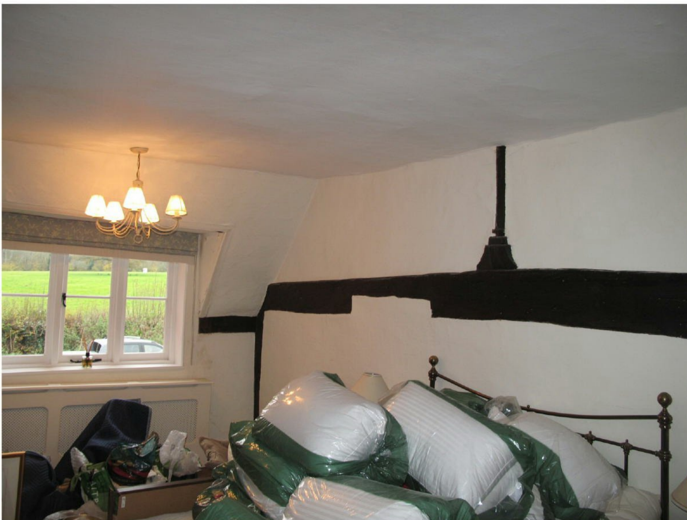
6. Ceiling finishes to be removed to investigate structure above
