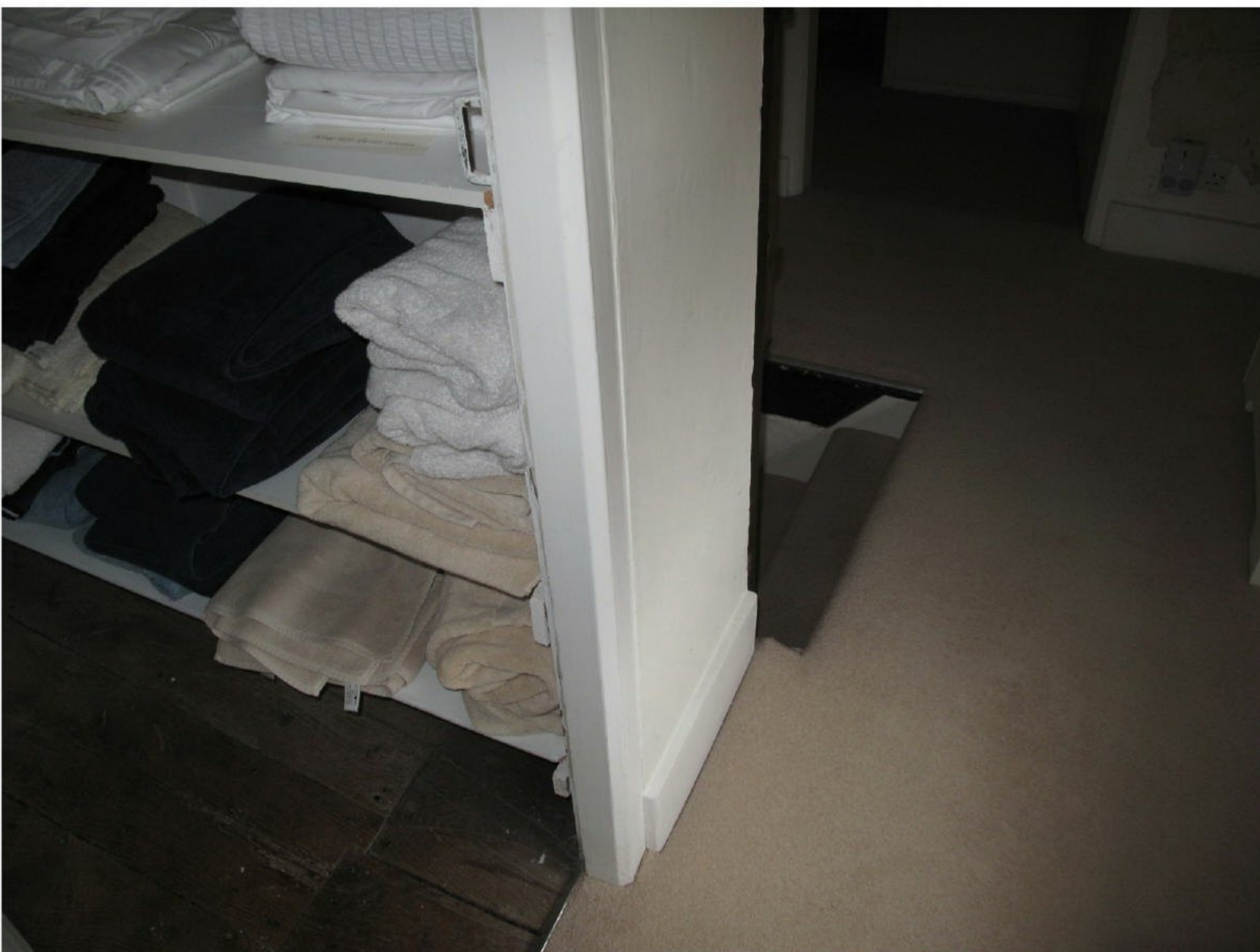
4. Stud wall removed and infill to floor where stair removed
