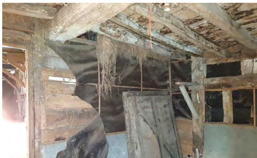
View 4: Looking northeast - historic boarded wall behind bituminous felt and battening (3.2.90*)
