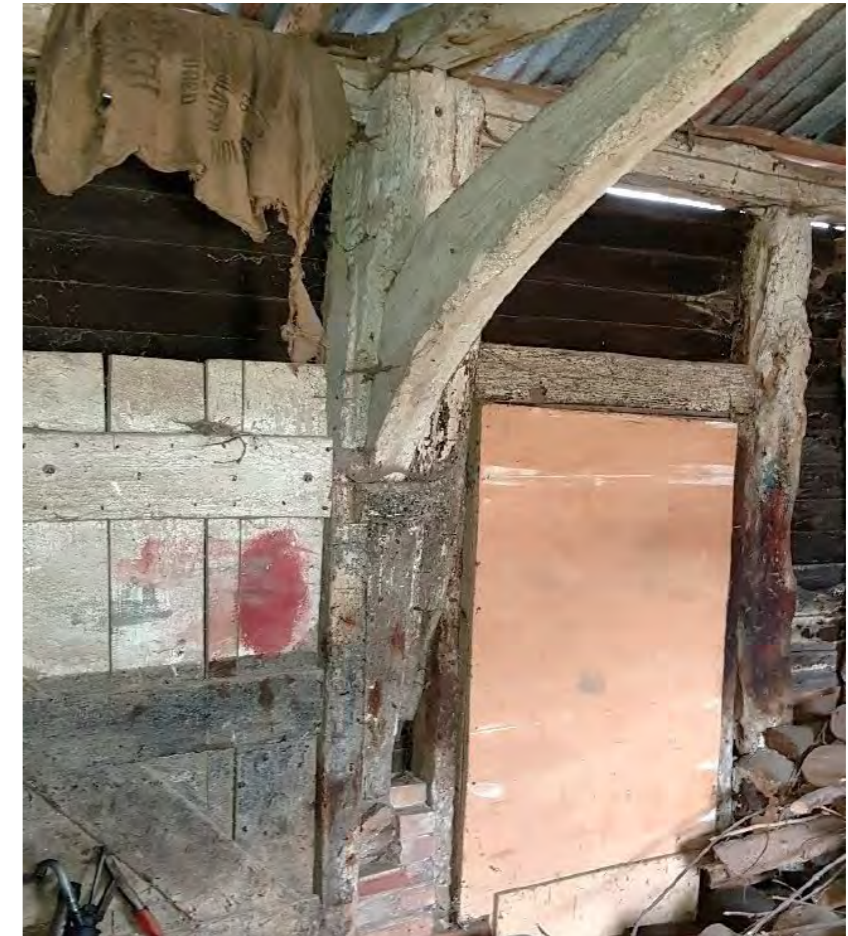
View 3: Looking east - existing single door opening (3.1.25*)
