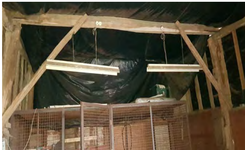
View 4: Looking south - sarking felt covering upper level
