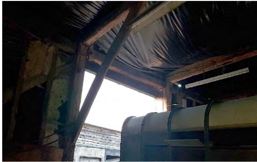
View 1: Looking west - Barn entrance (Bay 3), non-historic double door opening (3.2.60*)
