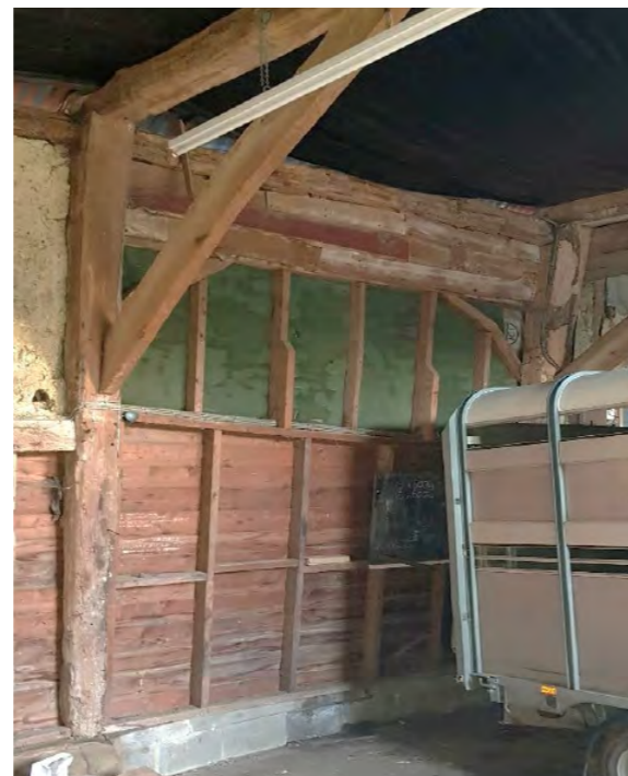
2 Bay 3 rebuilt and non-historic (3.2.40*)
