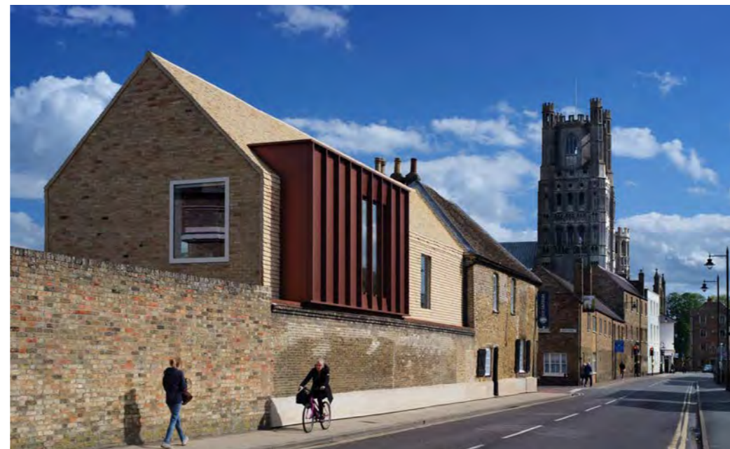
Ely Museum - restoration and extension of a Grade 2 listed building.
