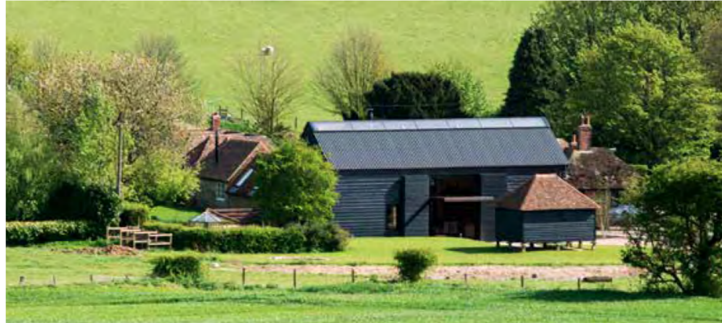
Timber framed barn has had a new steel and corrugated metal roof added with long linear rooflight
