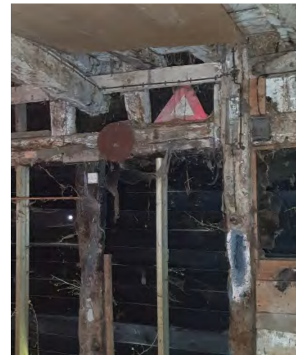
4 Exposed timber seen - elevation wrapped in a bituminous felt (3.2.77, 3.2.84*)
