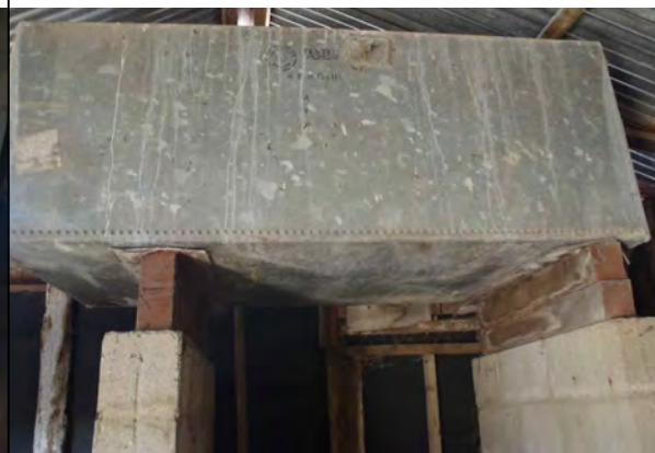
Photo 26 - Suspected water tank in Building 6
