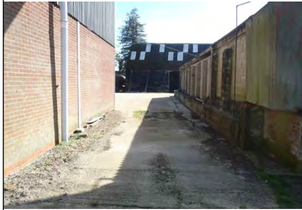
Photo 12 - Small retaining wall along the northern site boundary
