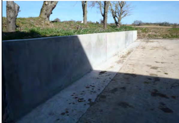
Photo 13 - Building 2, looking south-west
