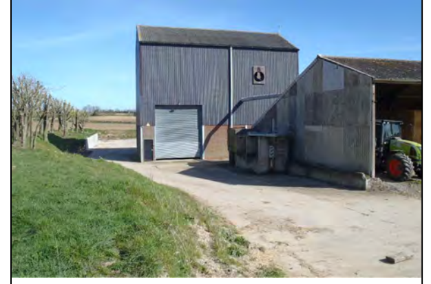
Photo 9 - Metal tanks to the north of Building 1
