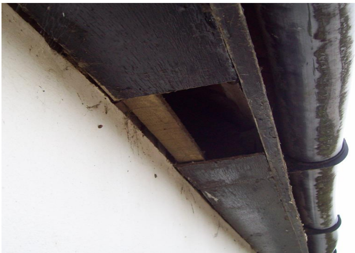
Plate 6: Detail of missing soffit board in B2.
