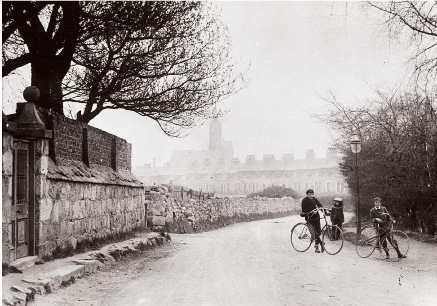
(Fig C2.01) Desswood Place was laid out in 1888 by the City of Aberdeen Land Association (CALA) in what was then a relatively rural area in the west end of Aberdeen but it was rapidly filled with large granite houses for the more prosperous citizens. The street was named after Alexander Davidson of Desswood who was Chairman of the Land Association for many years. Desswood was his country property near Kincardine O'Neil on Deeside. (Source: ACC Silver Vault)
