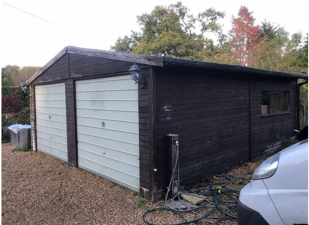
Existing timber clad garage to be replaced
