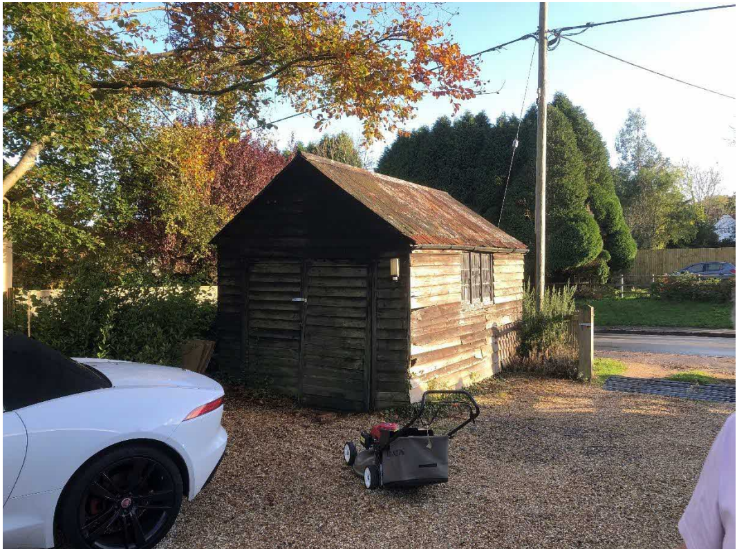
Existing shed alongside main road, to be replaced
