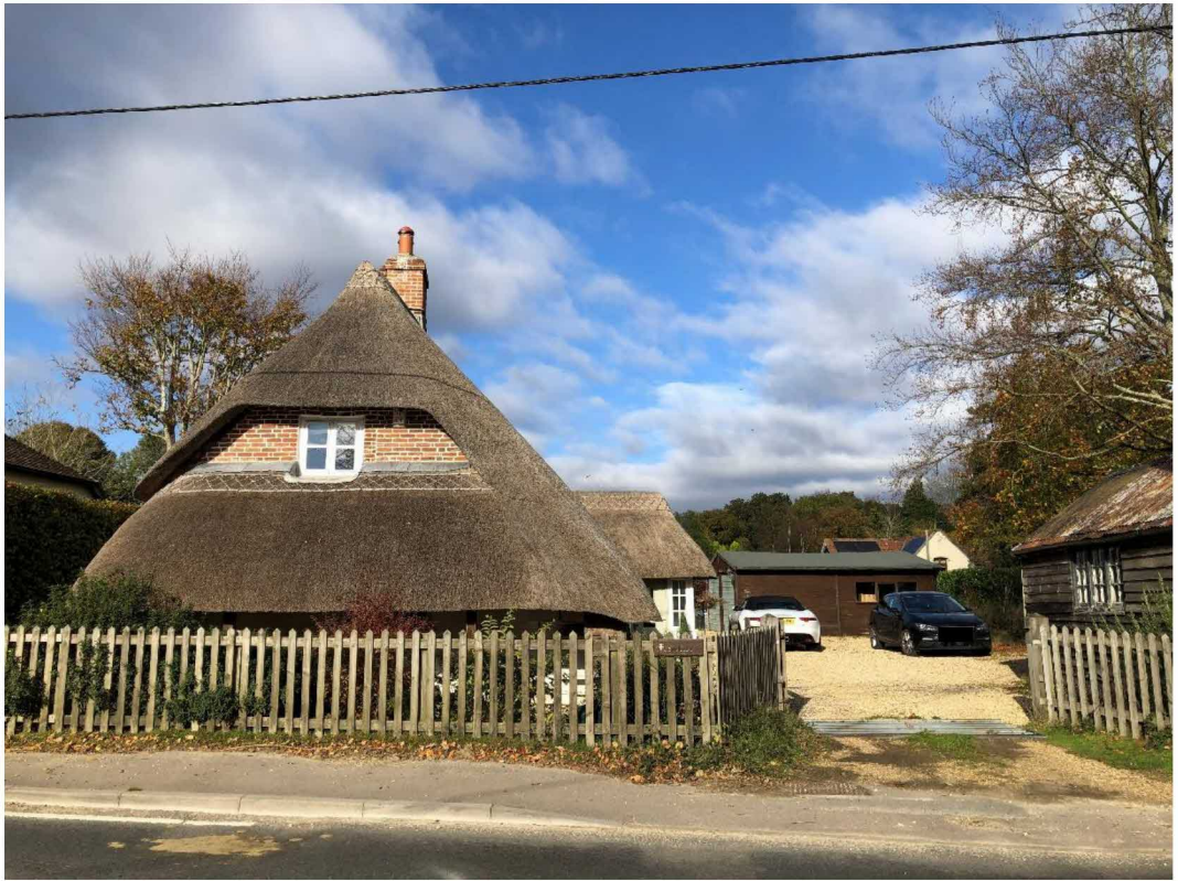
Elevation of Ramblers taken from main road with garage in distance, shed to right
